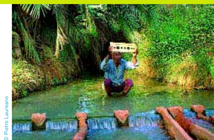
Photo 1. The foggaras system distributes water throughout the oasis.
