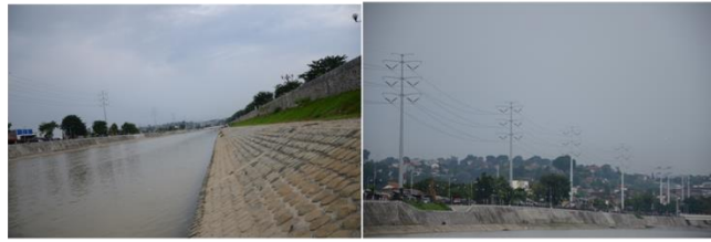
East Flood Canal
