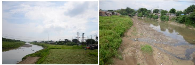
Figure 4 Existing Condition of Flood Canals in Semarang
