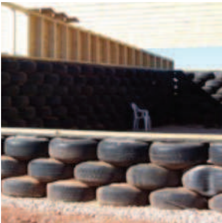
Tires - alternative foundation material similar to a retaining wall
