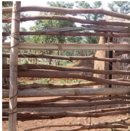
Small Sticks - form lath on which to apply mud
