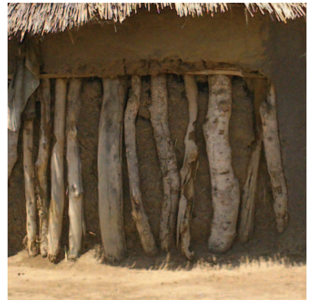
Large Branches - support roof structure
