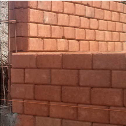
Machine made blocks - walls
