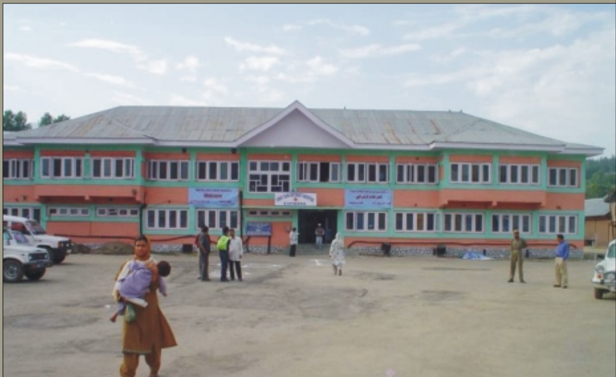
Repaired and Retrofitted Hospital after the 2005 Muzzafarabad Earthquake (M 7.6) Under guidance of Professor A. S. Arya
