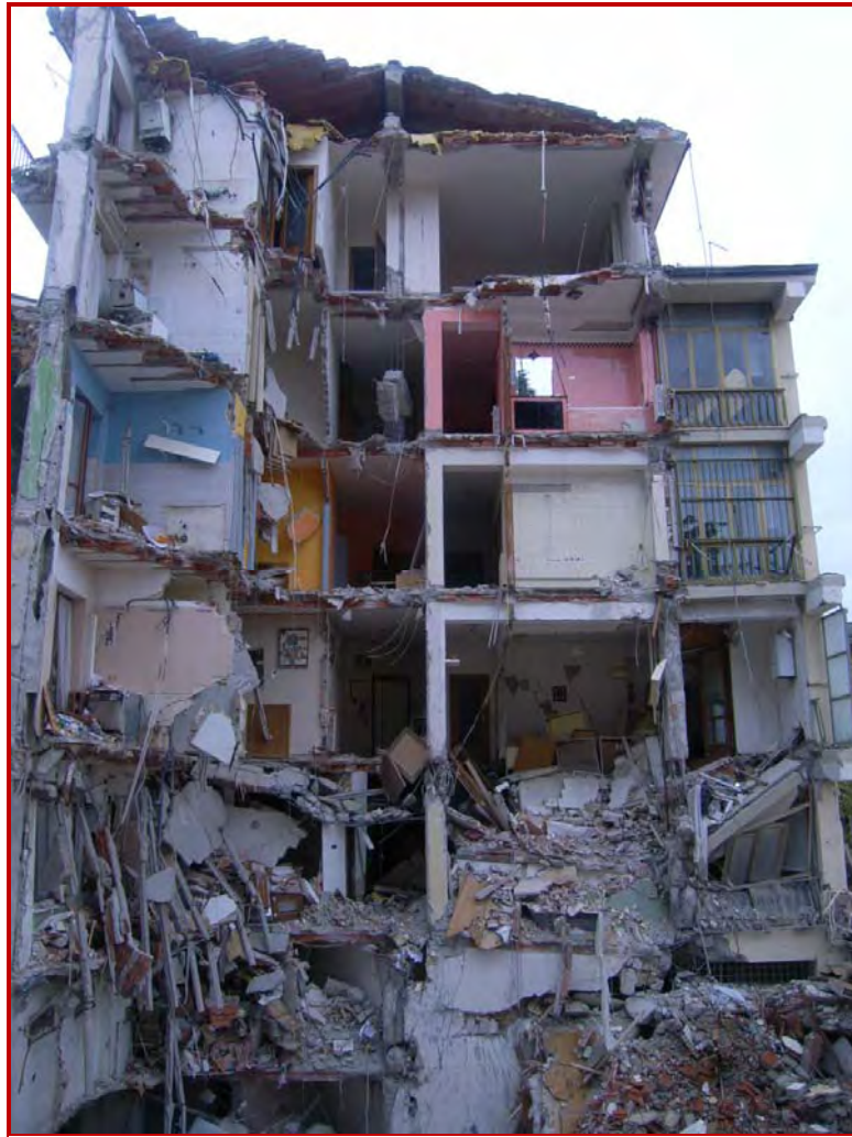
Figure 31: Residential building in Aquila on Via XX Settembre.
