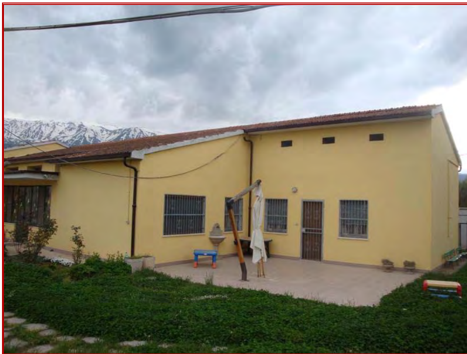
Figure 17: View of reinforced concrete frame with infill brick wall school building showing negligible damage.
