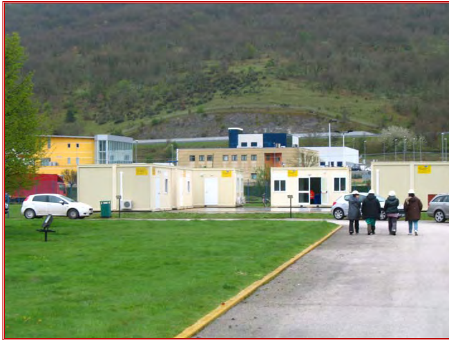
Figure 42: Temporary office housing in Dompe' Pharmaceutical Plant
