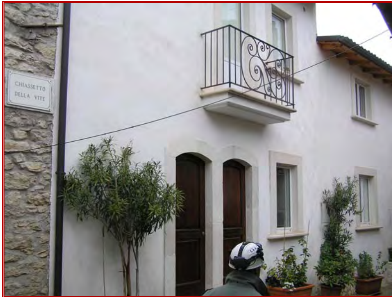
Figure 24: Recently restored masonry house in central Paganica that sustained no damage
