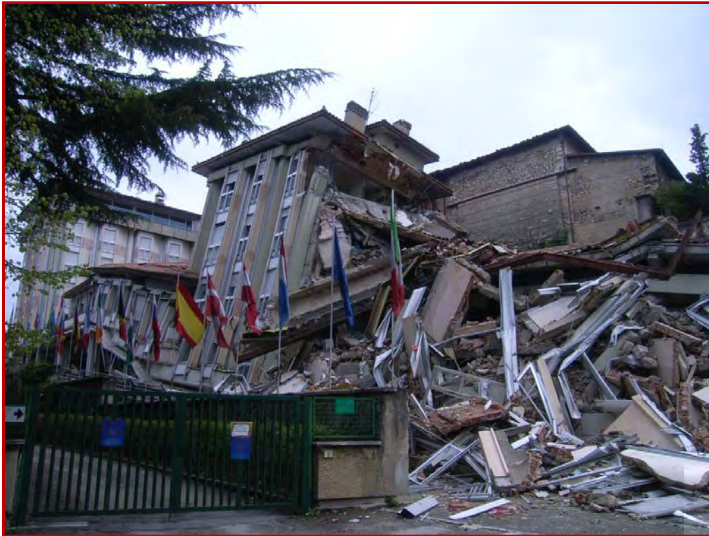
Figure 29: Hotel Degli Abruzzi in Aquila. Soft-storey failure of RC frame.
