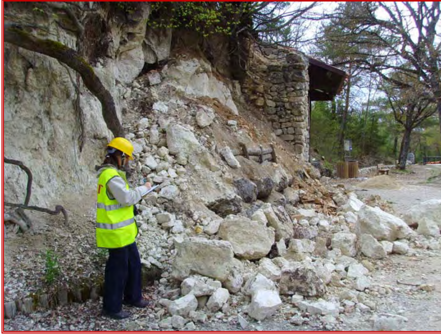
Figure 58: Rock fall at Lago Sinizzo
