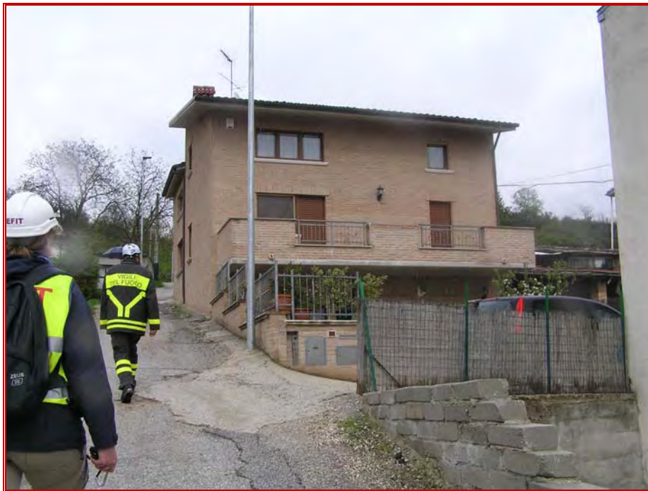
Figure 32: RC 2001 residential two-storey above Paganica Undamaged
