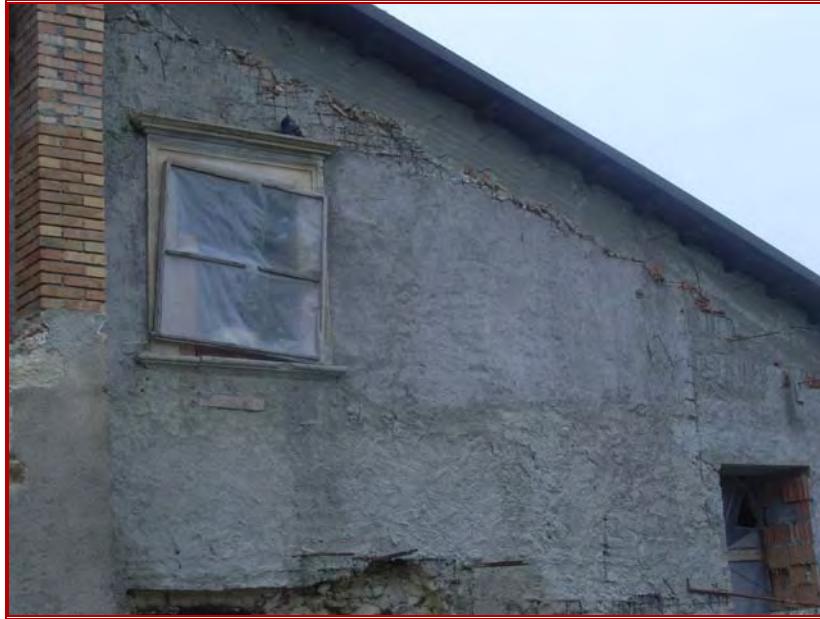
Figure 21: Masonry Structure in Process of Strengthening.
