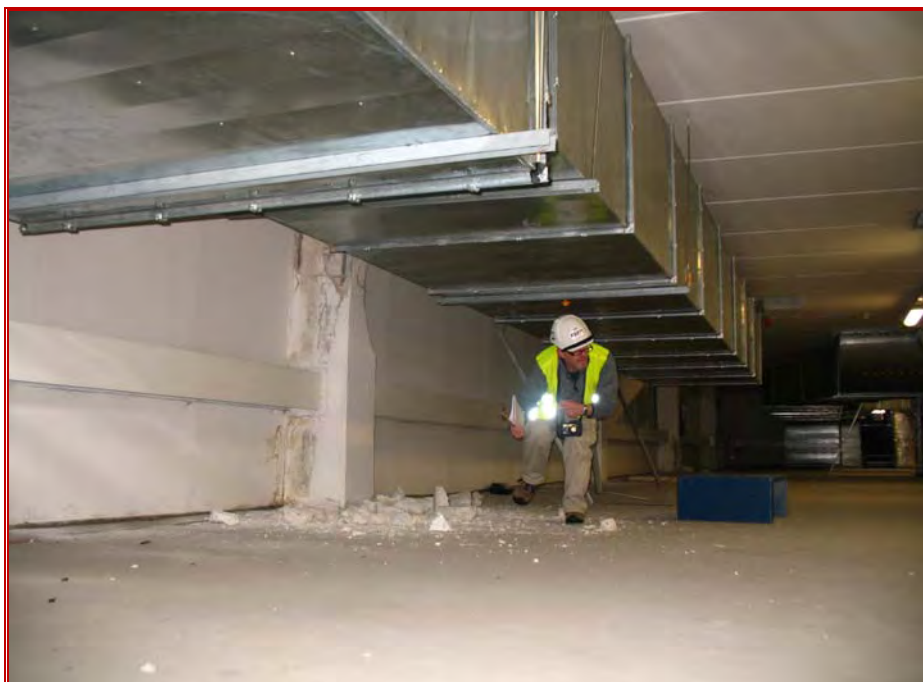
Figure 41: Short-column failure in Dompe' Pharmaceutical Plant
