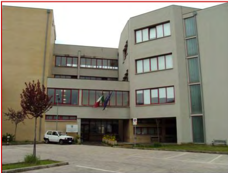
Figure 46. The Faculty of Medicine and Surgery building of Aquila University, located northwest of the Aquila hospital. The structure is formed of shear walls and withstood the earthquake without any visible damage.
