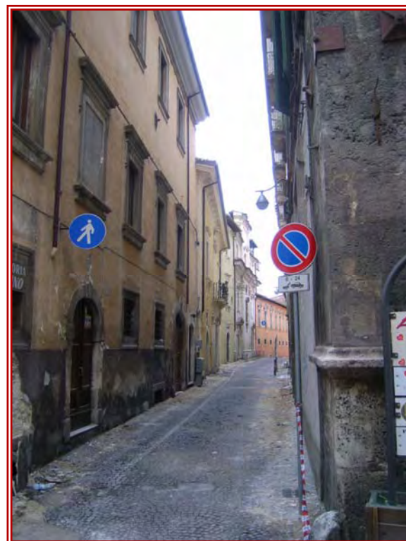
Figure 10: Typical residential street in the historic centre of L'Aquila flanked by 2-3 storey stone masonry buildings
