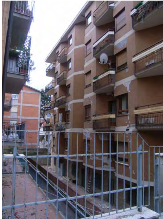
Figure 11: An example of a pre-1975 concrete frame reinforced concrete apartment block in L'Aquila, typically 5-8 storeys
