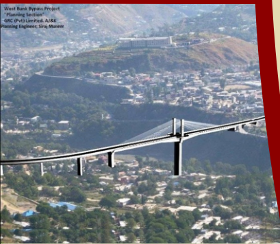
Naluchi Bridge, Muzaffarabad
