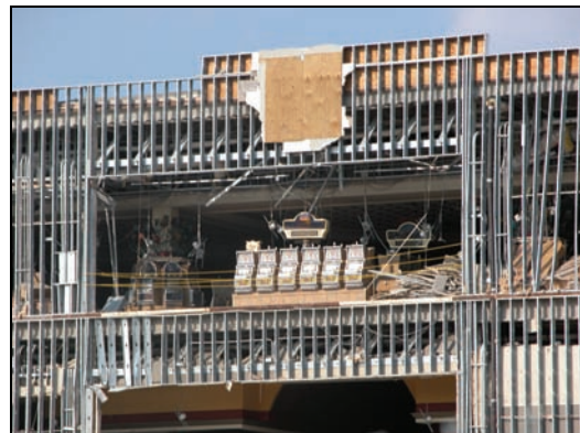
(b) Damage to Barge
