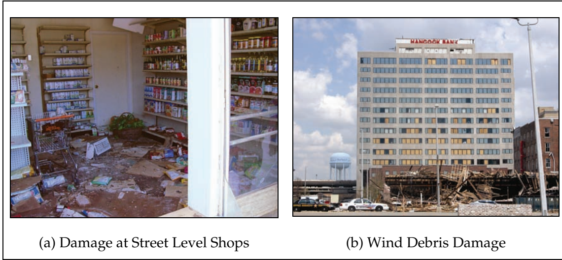
Figure 3-14. Flooding and wind damage in downtown Gulfport.
