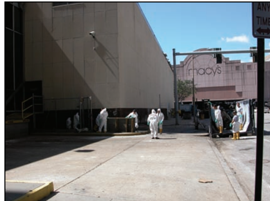
(b) Cleanup of Basement
