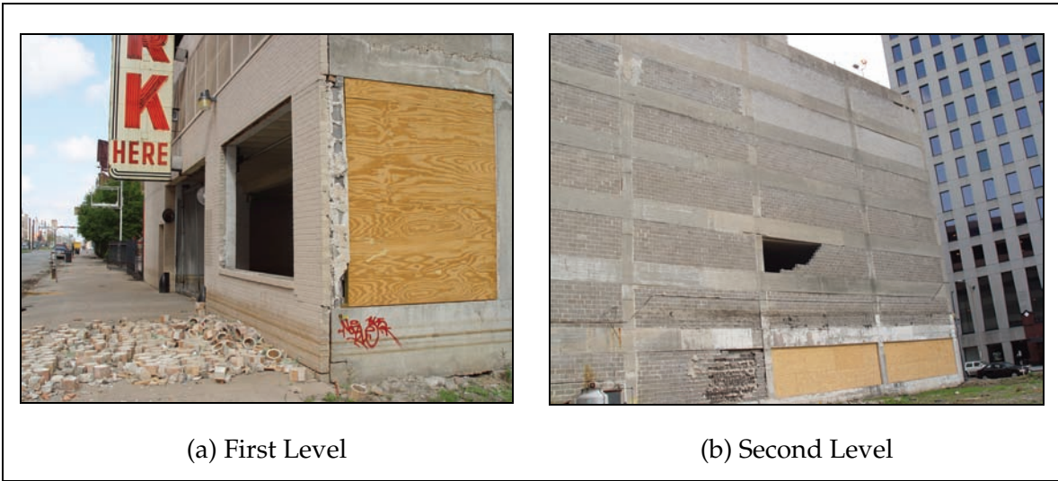
Figure 4-4. Masonry infill damage.
