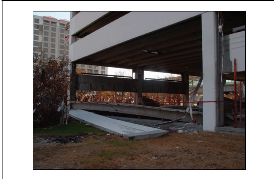
Figure 4-10. Flexibility of spandrel beams.
