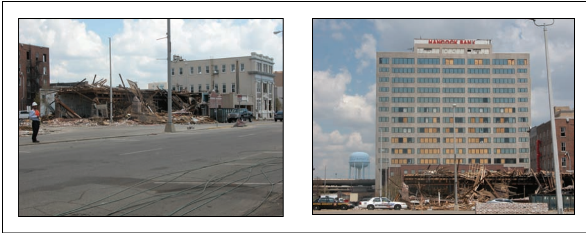
Figure 4-1. Left: partial collapse of unreinforced masonry bearing-wall building, downtown Gulfport MS. Debris from this building may have impacted a high-rise building downwind, causing extensive wind damage (right).
