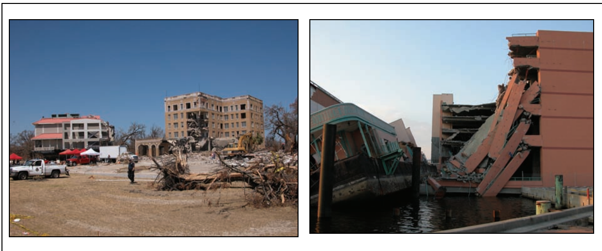
Figure 4-5. Structural damage resulting from surge-borne debris.
