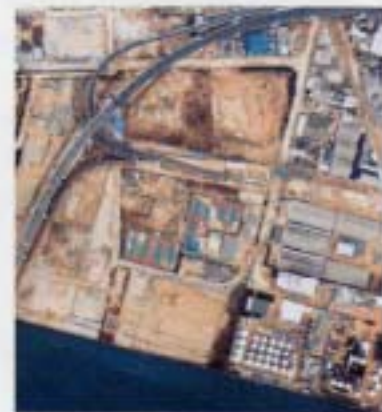
Aerial photograph of liquefaction that occurred during the Great Hanshin-Awaji Earthquake.
