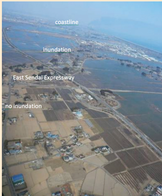
FIGURE 1: East Sendai Expressway
