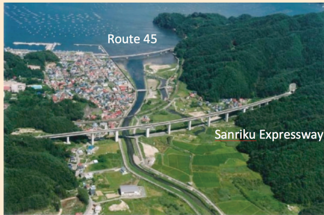
FIGURE 2: The Sanriku Expressway was built with tsunamis in mind
