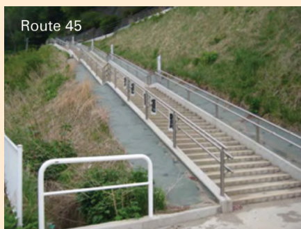
FIGURE 5: Evacuation stairway at the Omoto Elementary School
