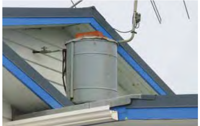
External header tanks can fall over in an earthquake and damage your water supply pipes, roof and guttering.
