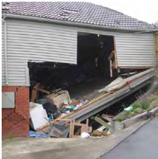
An example of floor support failure where the under floor framing has failed in an earthquake.
