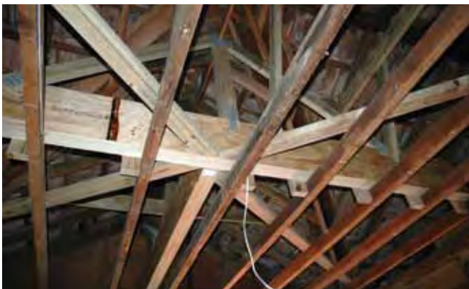
An example of additional roof bracing.
