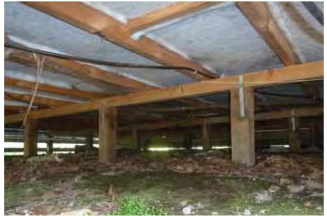
Unbraced pile foundations.
