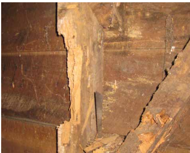
Borer beetle attack to wall framing timbers.
