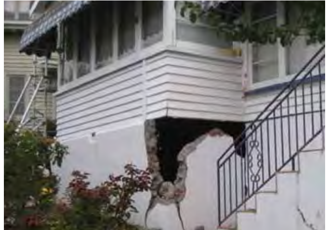
Unreinforced concrete foundations can fail in an earthquake.
