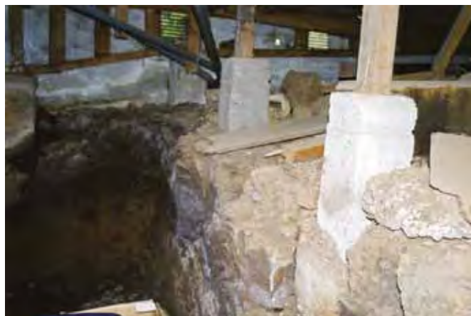
Pile support weakened by ground excavation.
