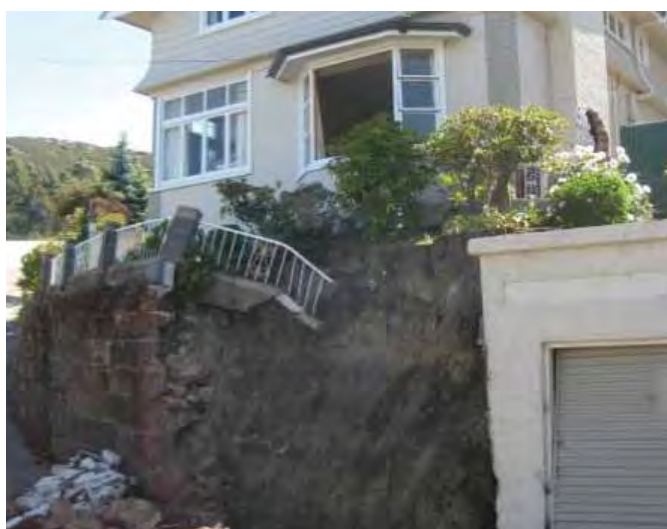
Unreinforced retaining wall collapsed in an earthquake.
