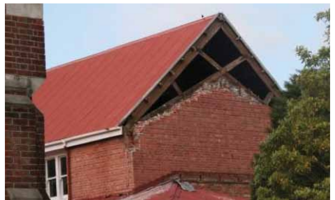
A double skin brick gable end. These are prone to damage in an earthquake.
