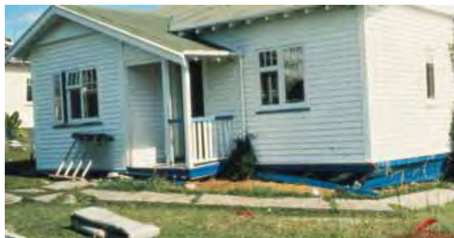
An example of a house that has slid off its foundations.
