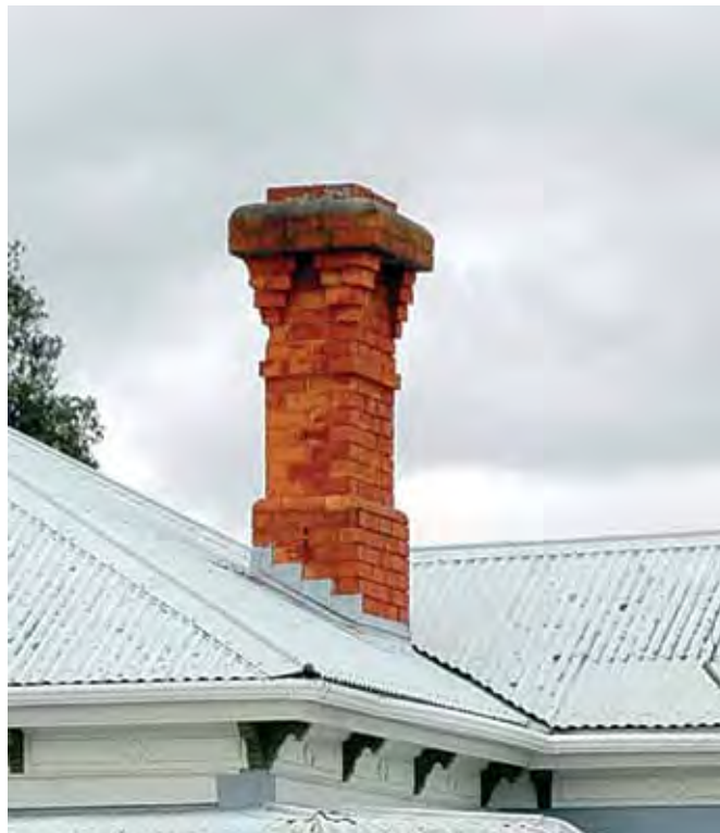
A typical unreinforced chimney found in many New Zealand houses.
