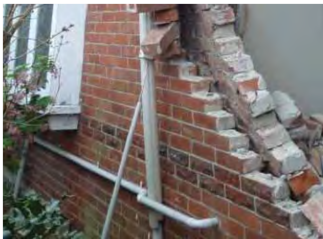
Double brick walls are prone to damage during an earthquake.
