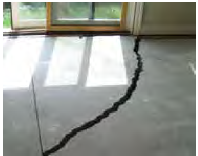
Unreinforced concrete slab foundations can crack in an earthquake if the ground spreads beneath the slab.
