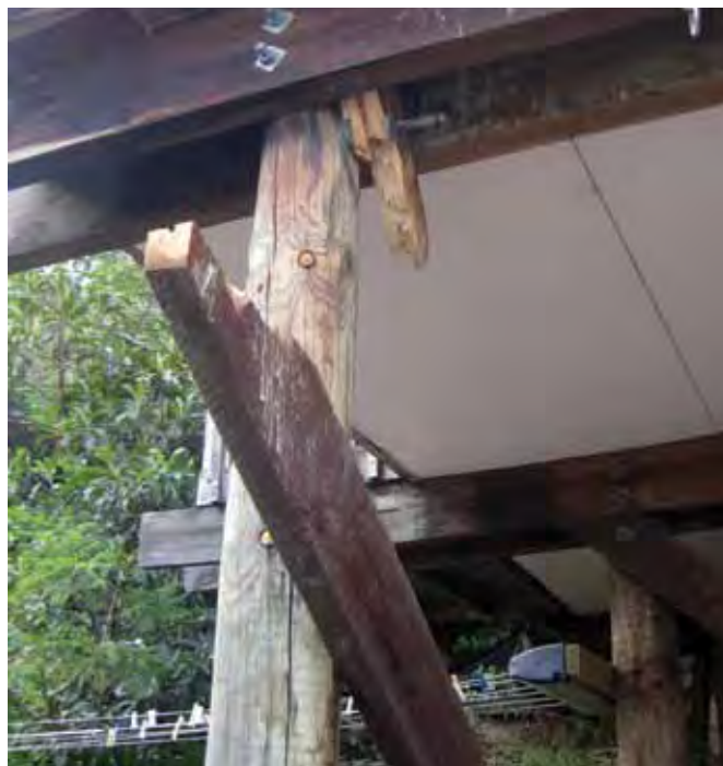
Foundation timber post and brace failure (the brace split in an earthquake because fixings were too close to the end).
