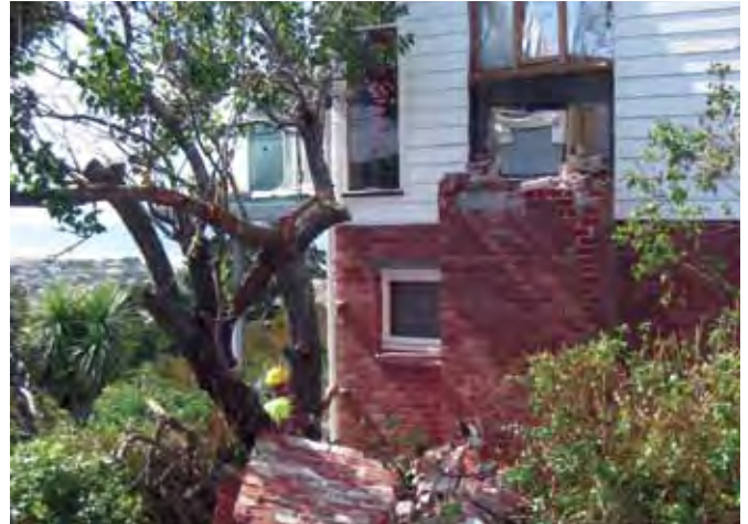
A house where the brick chimney has failed.
