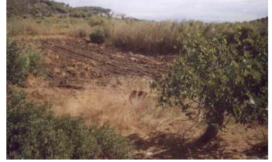
Marshy area on the E. part of Brauron site after clearance works (field visit of 24/09/2006)
