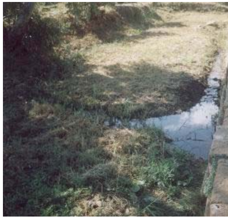
Stagnant waters in the subsided ground
