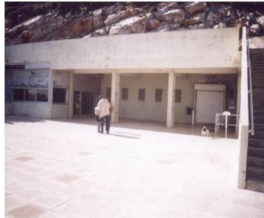
Koutouki cave. Entrance facilities Mountain Hymettos
