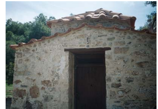
Byzantine church of Saint George – after restoration works
