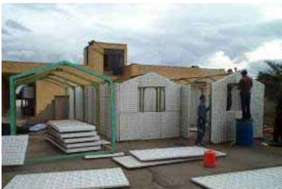
Temporary shelters in Bonyad Maskan office in Bam. Portal frames with prefabricated wire mesh panels are covered with layers of concrete from inside and outside.
