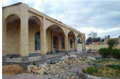
Housing and Urban Development Organisation's Bam office. Another masonry building with a jack-arch roof system and ties experiencing collapse of parapets and moderate damage inside the building.
