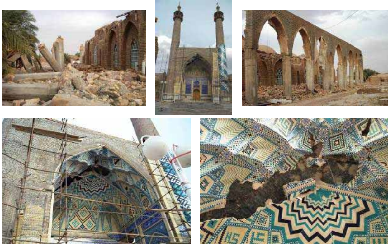
Figure 54: Emamzade Zied in Bam. Extensive damage to the sides of the main building which appear to be an extended part of an older section of the structure. The main building has not collapsed.
