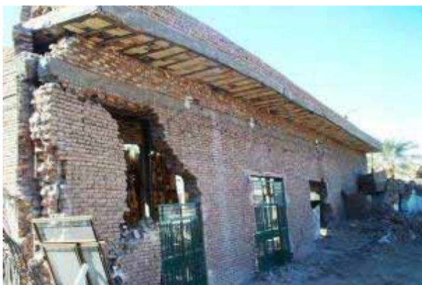
Front load bearing masonry wall
