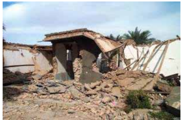
Figure 28: A residential masonry building without ties in Baravat in the same alleyway as Bagheri primary school in Figure 35. Construction finished about 6 months before the earthquake with a roof system of steel joists and brick arches with no structural system providing overall integrity. Heavy roof slippage over the walls resulted in collapse of walls and the whole structure. Poor materials and construction led to the collapse. The mortar used is lime-sand. Fortunately, the whole family escaped by being vigilant and sleeping outside after the initial pre-shock. Many other buildings of similar construction had completely collapsed in the same alleyway. Another example is shown in the lower right photograph.
