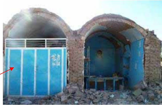
Local shop buildings in Bam, near to Emamzadeh Ali Ebn-Hassan, with a barrel vaulted roof system. The buildings are standing but all facades, made from fired bricks introduced later and covering the front of the thick walls and roof have separated from main mud brick structure and collapsed.
