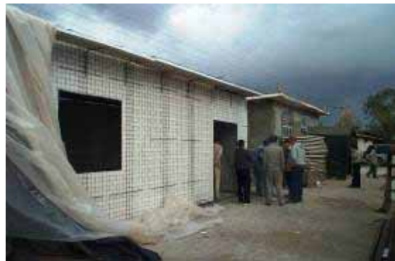
Another type of temporary shelter built using wire mesh panels and concrete cover
