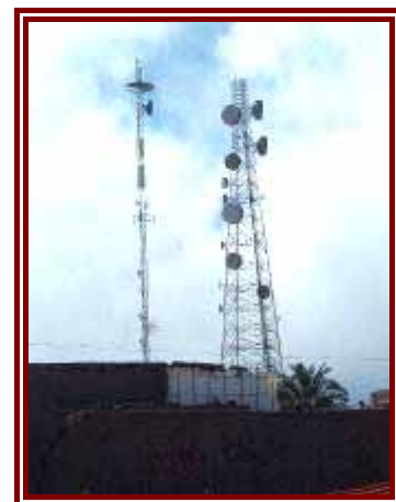
Figure 9: One of the main telecommunication towers in Bam which survived the earthquake
