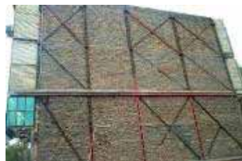
Figure 44: Good performance of some steel structures with a braced frame structural system opposite the Imam hospital in Bam (various views of the same building in each row, except lower row). Bracing in top left has buckled out of plane of the wall and detached from the top joint.
