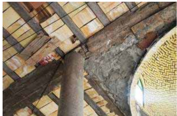
Concrete joist-hollow block roof
