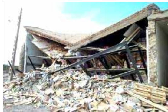
Figure 55: Khatam-Al Nabiein Cool Storage-North of Bam, located on the other side of the Posht Rod river across Bam's main bridge. The roof system is hollow bricks with reinforced concrete joists and slab. Internal steel frames providing shelving to the date packages were not properly designed for the heavy load of date packs. It is constructed from several independent two storey frames extending between the main walls with no positive connection tying them to each other or to the walls. The shelving floors are made from lumber, sitting on the steel beams. The shelving frame collapsed in its weaker out of plane direction due to inertia forces from the earthquake. The collapse of these shelving frames removed the support from the front of the building and resulted in building collapse.
