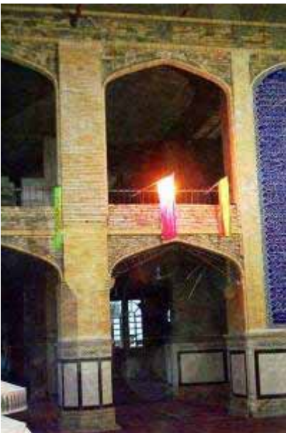
Figure 51: Jame Mosque in Bam. Reinforced concrete frame with joist and hollow brick RC slab roof and masonry infill walls. The central dome has a steel frame structure and is built from fired bricks. No sign of significant damage either on the interior or on the exterior of the structure or minarets.
