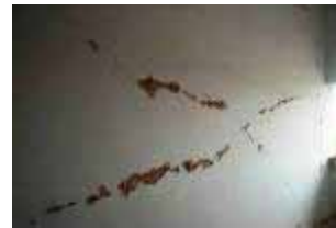
Separation of tiles in stairs
