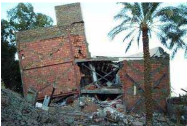
View from the south
