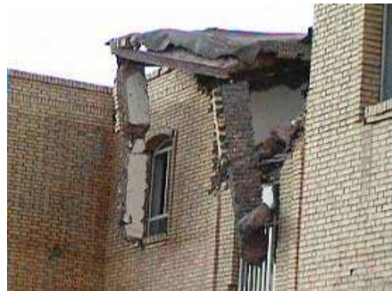
Figure 58: Examples of the performance of staircase extension structures in Bam Earthquake for Masonry buildings: Housing and Urban Development Organization’s new ‘build to rent’ project. There were a large number of collapsed staircase extension structures in this project, only some examples are shown here.
