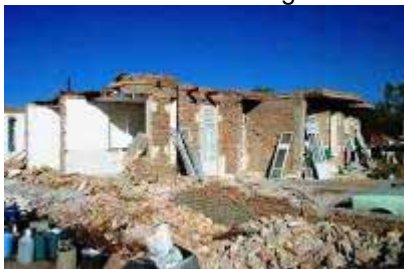
A masonry building in Bam incorporating vertical and horizontal ties but with poor concrete quality.
