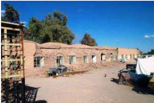
Another example of adobe building with double spanned vaulted roof, standing after the earthquake showing damage to the fired brick facade
