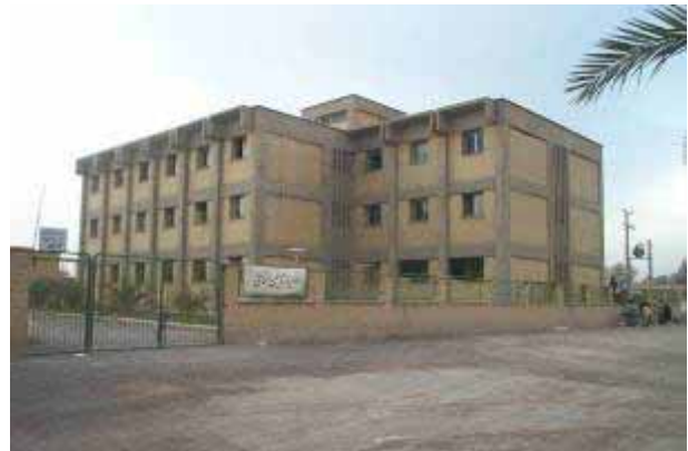
Undamaged in a reinforced concrete building
