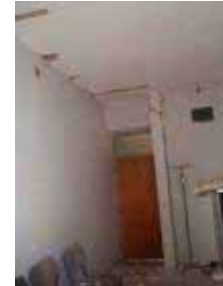
Housing and Urban Development Organisation's Bam office. Another masonry building with a jack-arch roof system and ties experiencing collapse of parapets and moderate damage inside the building.
