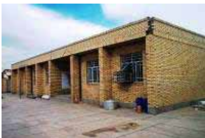
Figure 35: Bagheri Primary School in Baravat, One storey masonry building with ties. Standing without major damage. Parapets at the back of the building and a part of the surrounding wall have collapsed due to collapse of a building on the other side of the wall. Minor damage on inside walls.
