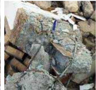
Details of poor materials and workmanship
