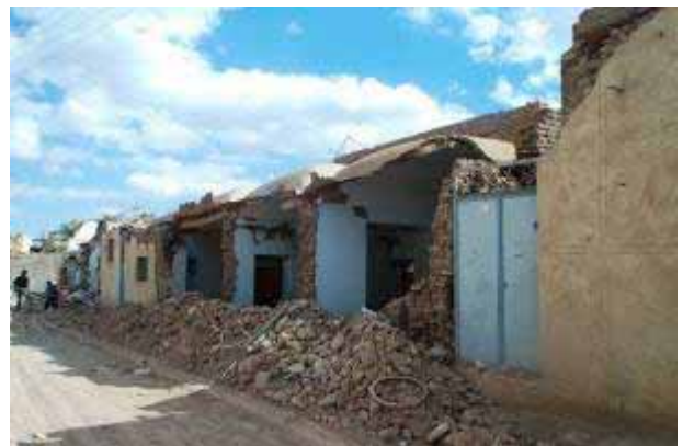
Figure 22: Bam's old district, examples of total collapse of mud-brick buildings
