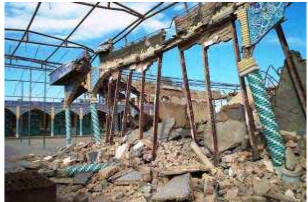
Figure 52: Mausoleum of Emamzadeh Ali Ebn Al-Hossain In Bam. Complete collapse of the main dome and its supporting old walls in the interior part of the mausoleum. These walls were mainly made from mud bricks. A steel frame envelops the building with a jack-arch roof system extending from the frame to interior masonry walls. The collapse of the main building appears to be the main cause of damage to the roof and external frame.
