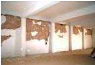
Inside view on upper floor showing collapse of infill wall next to a door opening
