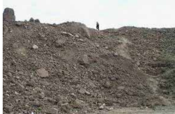
West wall from outside
