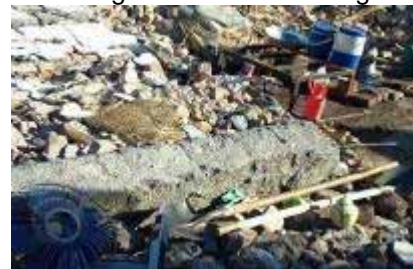
A masonry building in Bam incorporating vertical and horizontal ties but with poor concrete quality.
