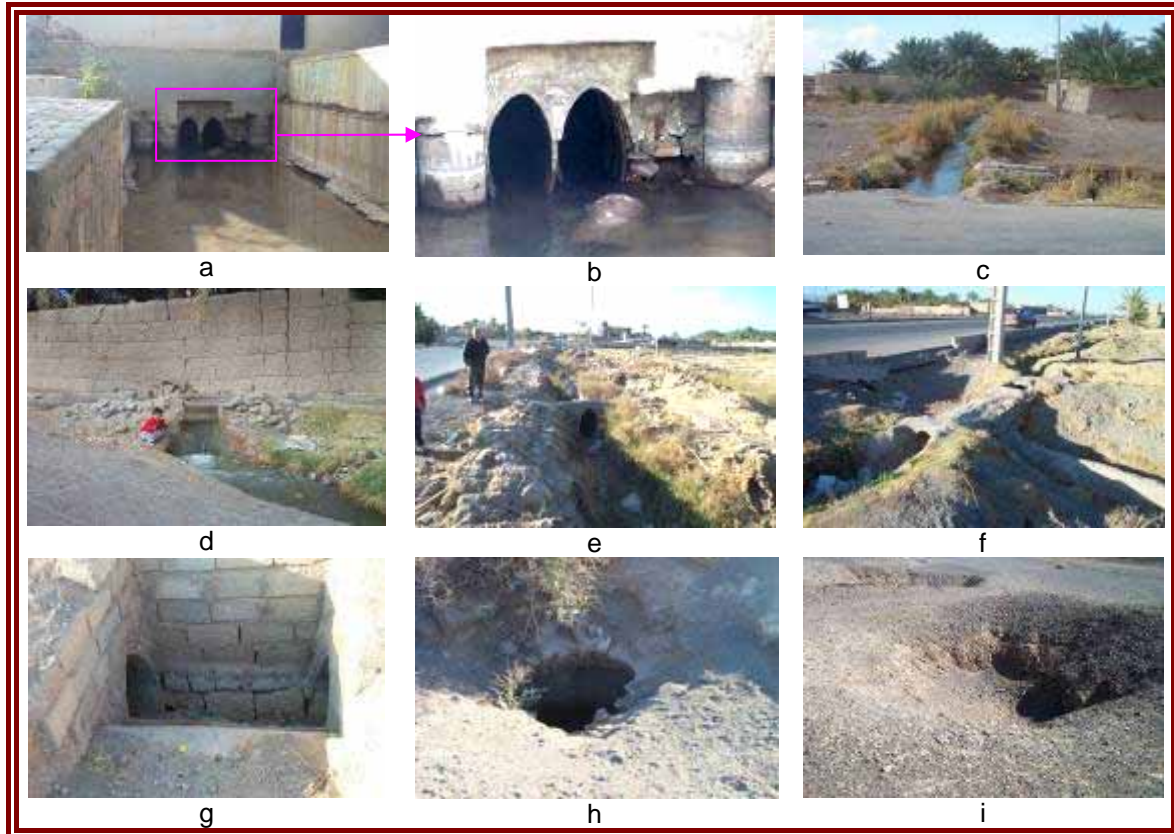
Figure 12: (a,b) An active qanat in Bam city showing the outlet below a residential building standing after the earthquake (c,d) an active qanat in Nartij village, northeast of Bam, (e-h) A dried qanat in Baravat with outlet to an open channel, distribution point, access facility at street level and the access shaft further up in a nearby field (i) Access Shaft for an old qanat near Nartij Village
