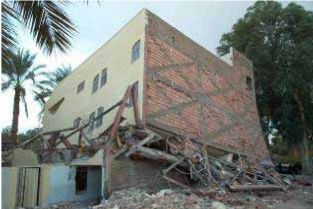
View from north-east
