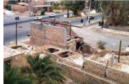
A masonry building in Baravat under construction. No vertical ties at the first storey were observed
