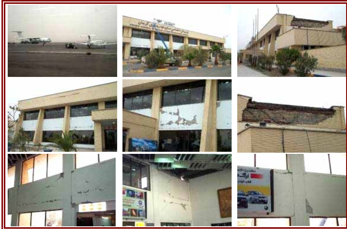
Figure 8: Bam Airport: Damage to the airport building in form of cracks and partial failure of non-structural fixtures. The first two rows show views from the outside of the building with the bottom row showing the inside of the building.
