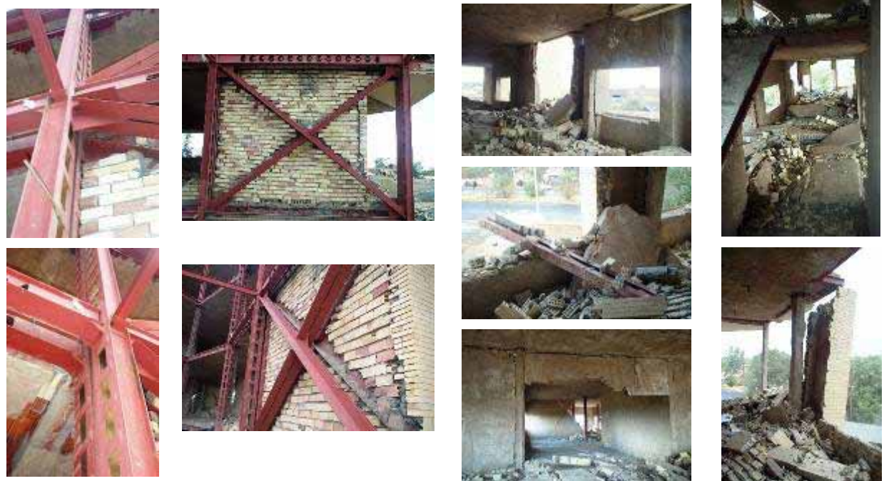
Some details of steel frame
