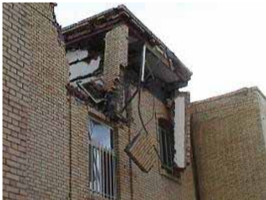
Figure 58: Examples of the performance of staircase extension structures in Bam Earthquake for Masonry buildings: Housing and Urban Development Organization’s new ‘build to rent’ project. There were a large number of collapsed staircase extension structures in this project, only some examples are shown here.
