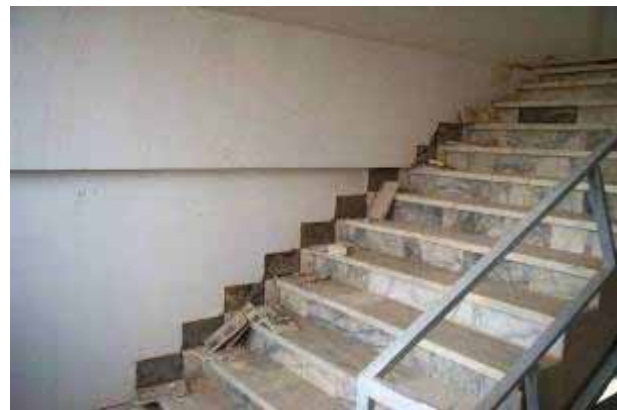
Separation of tiles in stairs
