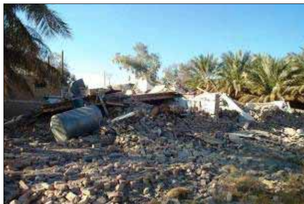
Figure 31: Kharazmi High school in Bam. Masonry building with a jack-arch roof system without ties that suffered total collapse.
