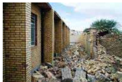
Figure 35: Bagheri Primary School in Baravat, One storey masonry building with ties. Standing without major damage. Parapets at the back of the building and a part of the surrounding wall have collapsed due to collapse of a building on the other side of the wall. Minor damage on inside walls.
