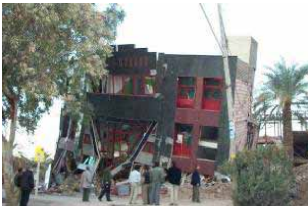
View from the west
