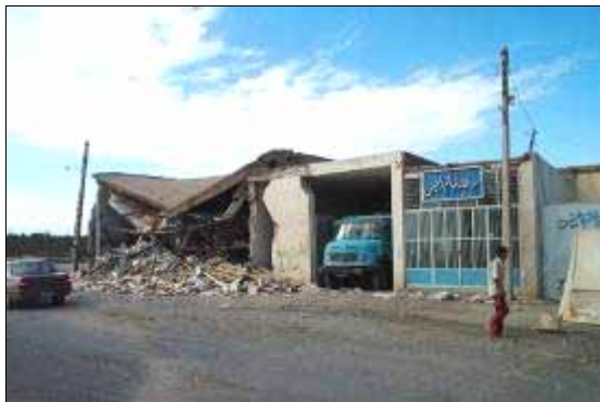
Figure 54: Emamzade Zied in Bam. Extensive damage to the sides of the main building which appear to be an extended part of an older section of the structure. The main building has not collapsed.
