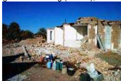
A masonry building in Bam incorporating vertical and horizontal ties but with poor concrete quality.
