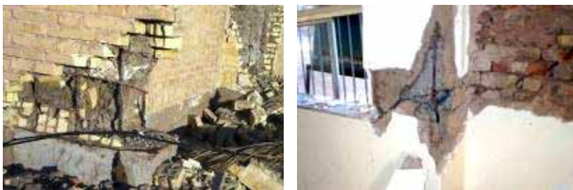
Details showing the poor concrete quality in vertical RC ties and generally bad workmanship
