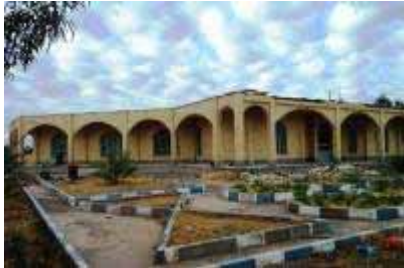
Housing and Urban Development Organisation's Bam office. Another masonry building with a jack-arch roof system and ties experiencing collapse of parapets and moderate damage inside the building.
