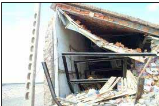
Figure 55: Khatam-Al Nabiein Cool Storage-North of Bam, located on the other side of the Posht Rod river across Bam's main bridge. The roof system is hollow bricks with reinforced concrete joists and slab. Internal steel frames providing shelving to the date packages were not properly designed for the heavy load of date packs. It is constructed from several independent two storey frames extending between the main walls with no positive connection tying them to each other or to the walls. The shelving floors are made from lumber, sitting on the steel beams. The shelving frame collapsed in its weaker out of plane direction due to inertia forces from the earthquake. The collapse of these shelving frames removed the support from the front of the building and resulted in building collapse.
