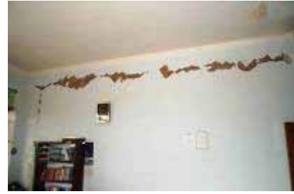
Bonyad-Shahid masonry office building in Bam showing damage to parapets and inside the building. Overall moderate damage
