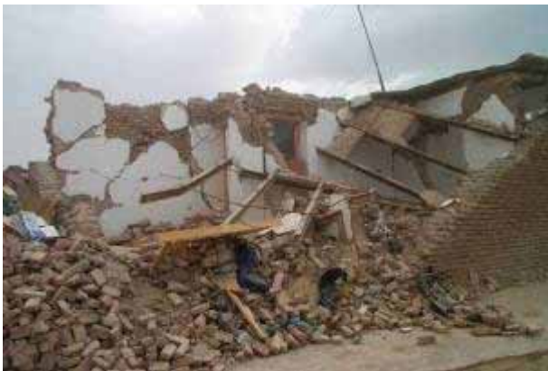
Figure 28: A residential masonry building without ties in Baravat in the same alleyway as Bagheri primary school in Figure 35. Construction finished about 6 months before the earthquake with a roof system of steel joists and brick arches with no structural system providing overall integrity. Heavy roof slippage over the walls resulted in collapse of walls and the whole structure. Poor materials and construction led to the collapse. The mortar used is lime-sand. Fortunately, the whole family escaped by being vigilant and sleeping outside after the initial pre-shock. Many other buildings of similar construction had completely collapsed in the same alleyway. Another example is shown in the lower right photograph.
