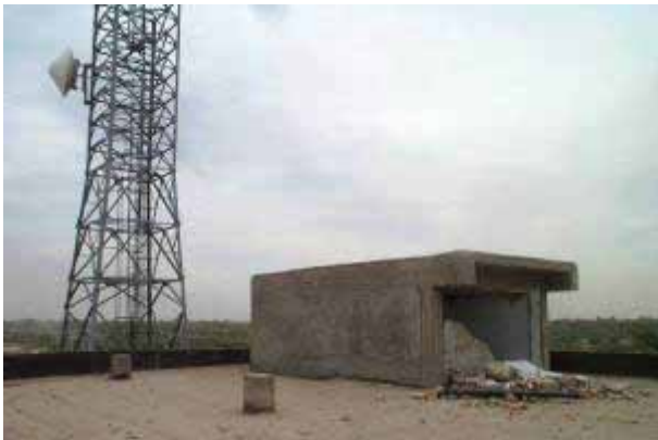
Baravat Telecommunication office
