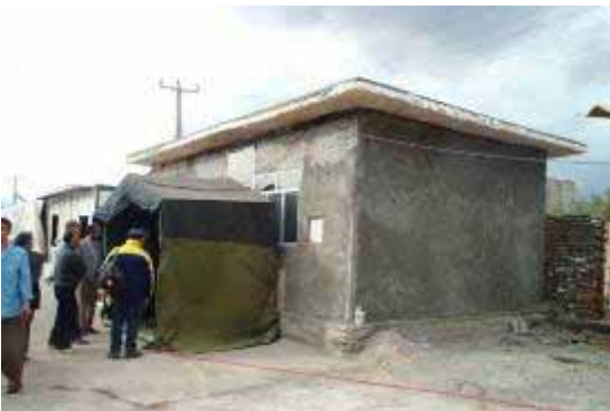
Another type of temporary shelter built using wire mesh panels and concrete cover
