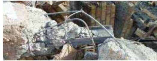
Details of poor materials and workmanship
