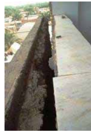
Separation of the facade from the wall below a window
