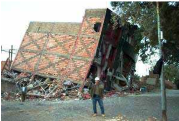
View from the north-west
