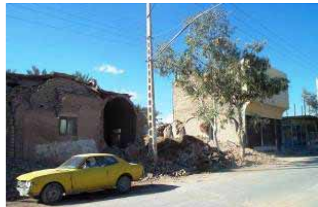
Figure 25: Damage to adobe buildings in contrast to other types of construction in the old district of Bam (left: a modern masonry building standing without major damage. Right: a steel structure with braced frame system with minor non-structural damage).
