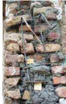
Details of poor materials and workmanship
