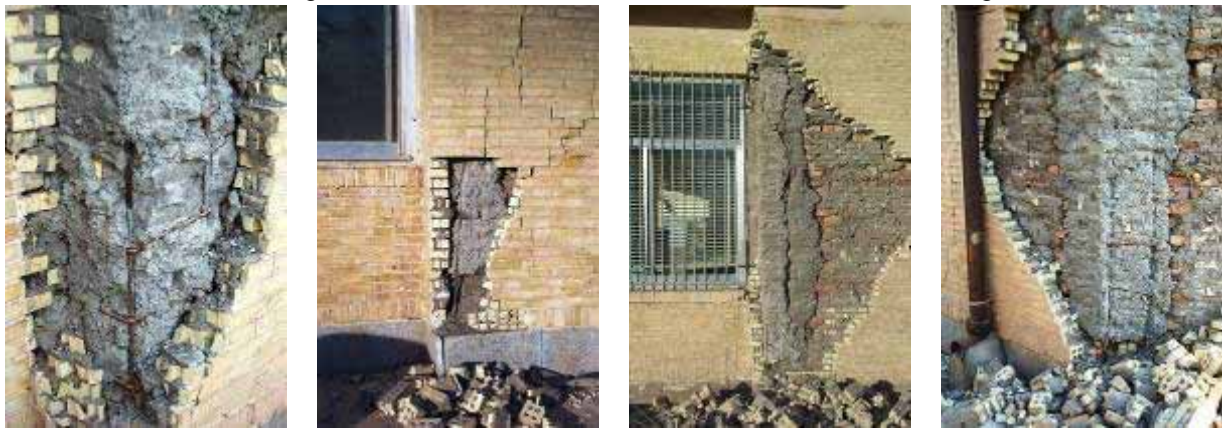
Details showing the poor concrete quality in vertical RC ties and generally bad workmanship
