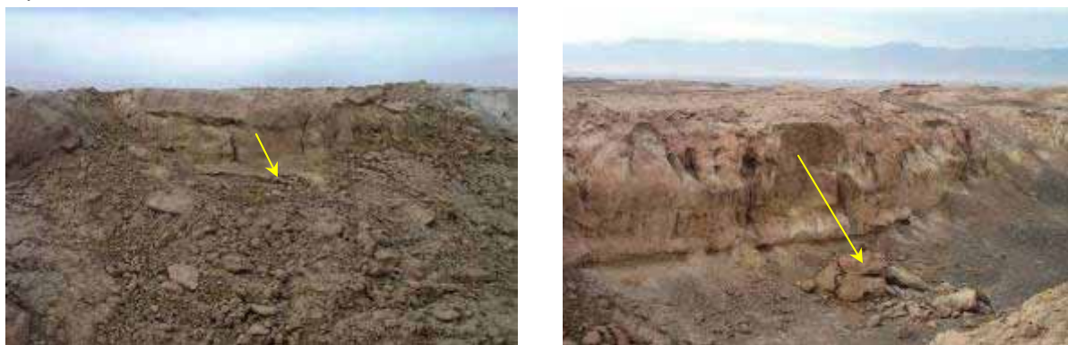
Figure 13: A minor landslide and a fall in southeast of Bam, near to the Bam-Baravat main road
