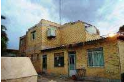
Governor's office building in Bam. Masonry with horizontal ties, Apparently no vertical ties had been used in this building. Bam's accelerometer was based in this building before the earthquake.
