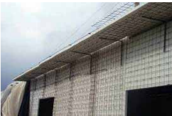
Another type of temporary shelter built using wire mesh panels and concrete cover
