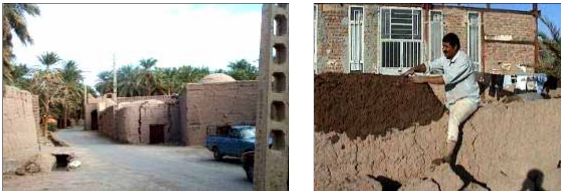
“ Chineh ” walls as part of courtyard wall (left) or bearing wall for houses (middle), Nartij Village
