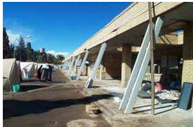
Figure 49: Imam Hospital in Bam, a single storey masonry building with a jack-arch roof system and inclined steel columns on the perimeter. Most of the building collapsed or was severely damaged. The Accident and Emergency Building collapsed due to the disproportionately thick and heavy roof, that buckled the external wall (left in 1 st and 2 nd row). Three roof insulation layers can be seen (3 rd row left).
