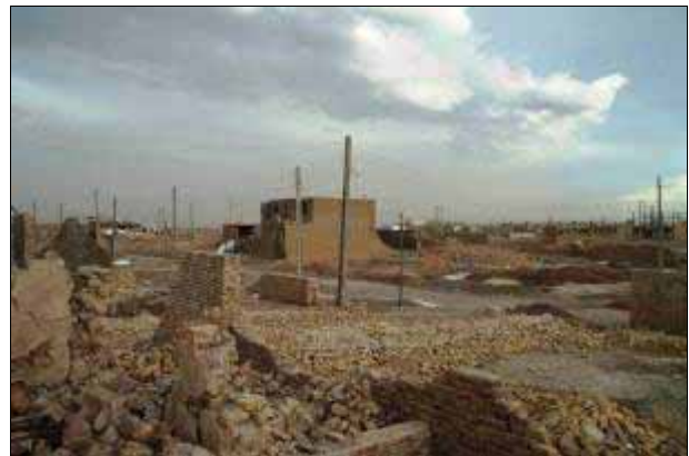
Figure 30: Razmandegan district of Bam. All the buildings in the district had recently been constructed, most of them consisting of masonry buildings with a jack-arch roof system without any ties. The majority of the buildings collapsed. In the building that can be seen standing in lower right corner photograph, horizontal ties could be clearly seen. This shows how proper construction practice could have made a difference to the outcome of this earthquake.
