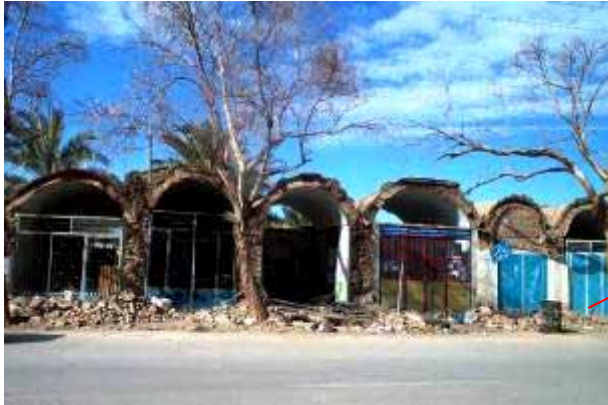
Local shop buildings in Bam, near to Emamzadeh Ali Ebn-Hassan, with a barrel vaulted roof system. The buildings are standing but all facades, made from fired bricks introduced later and covering the front of the thick walls and roof have separated from main mud brick structure and collapsed.
