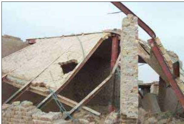
Figure 30: Razmandegan district of Bam. All the buildings in the district had recently been constructed, most of them consisting of masonry buildings with a jack-arch roof system without any ties. The majority of the buildings collapsed. In the building that can be seen standing in lower right corner photograph, horizontal ties could be clearly seen. This shows how proper construction practice could have made a difference to the outcome of this earthquake.
