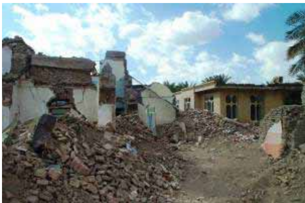
Figure 25: Damage to adobe buildings in contrast to other types of construction in the old district of Bam (left: a modern masonry building standing without major damage. Right: a steel structure with braced frame system with minor non-structural damage).
