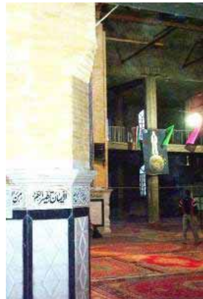
Figure 51: Jame Mosque in Bam. Reinforced concrete frame with joist and hollow brick RC slab roof and masonry infill walls. The central dome has a steel frame structure and is built from fired bricks. No sign of significant damage either on the interior or on the exterior of the structure or minarets.
