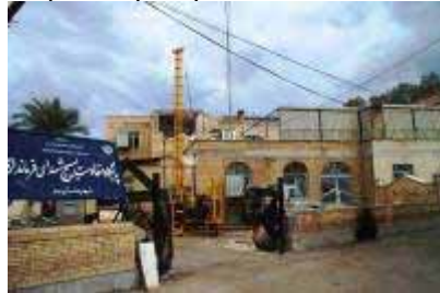
Governor's office building in Bam. Masonry with horizontal ties, Apparently no vertical ties had been used in this building. Bam's accelerometer was based in this building before the earthquake.
