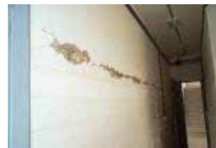
Separation of the facade from the wall below a window
