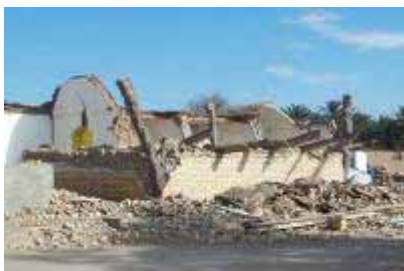
Esfikan Guidance school with 3 separate masonry buildings incorporating horizontal and vertical ties. One building completely collapsed (left) with the vertical ties standing and separated from the collapsed walls. Two other buildings are damaged but standing (middle), the internal damage is shown on the right.
