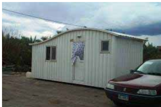
Prefabricated temporary shelter
