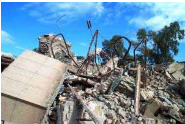
Figure 52: Mausoleum of Emamzadeh Ali Ebn Al-Hossain In Bam. Complete collapse of the main dome and its supporting old walls in the interior part of the mausoleum. These walls were mainly made from mud bricks. A steel frame envelops the building with a jack-arch roof system extending from the frame to interior masonry walls. The collapse of the main building appears to be the main cause of damage to the roof and external frame.
