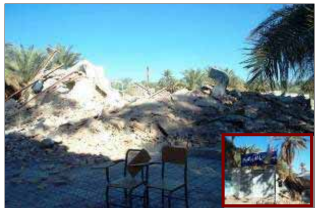
Figure 31: Kharazmi High school in Bam. Masonry building with a jack-arch roof system without ties that suffered total collapse.
