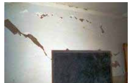
Figure 35: Bagheri Primary School in Baravat, One storey masonry building with ties. Standing without major damage. Parapets at the back of the building and a part of the surrounding wall have collapsed due to collapse of a building on the other side of the wall. Minor damage on inside walls.
