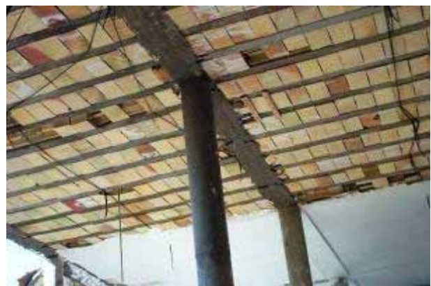
Concrete joist-hollow block roof
