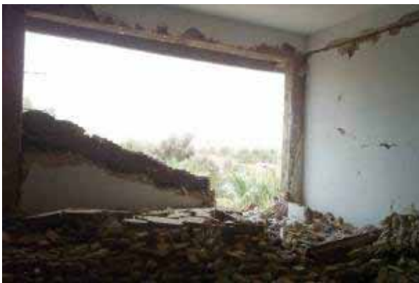
Inside view on upper floor showing collapse of infill wall next to a door opening
