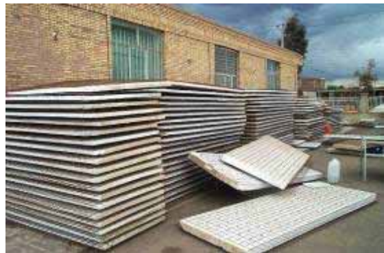
Temporary shelters in Bonyad Maskan office in Bam. Portal frames with prefabricated wire mesh panels are covered with layers of concrete from inside and outside.
