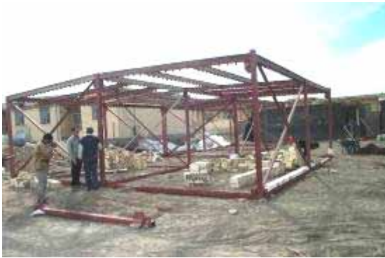
Steel frame temporary shelter is tested on-site in Baravat at the time of visit. No foundation was used for these test shelters. The roof system appears to be designed for a composite slab system. Some of the shelters at the back of the picture are shown covered by tent cloths.
