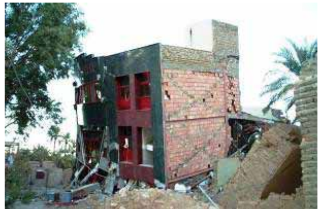
View from the south-east
