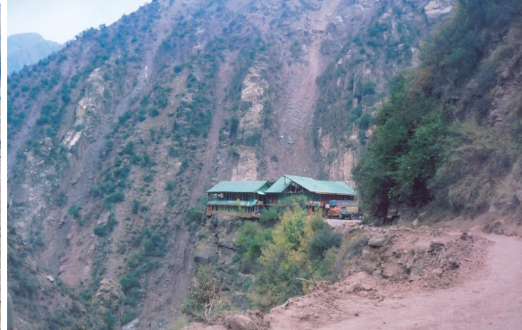
Buildings on the bed rock near Red Bridge, Uri
