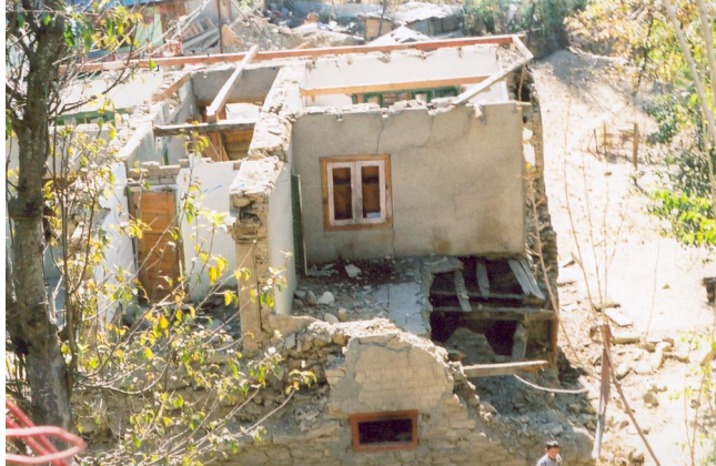
The inner walls intact in a mud mortar house (Karnah)
