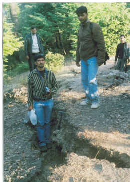
Fissures in the Green Patch Mountain
