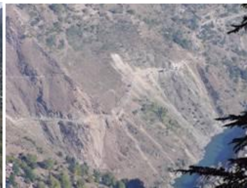
Landslides on the PAK Neelam Valley Road
