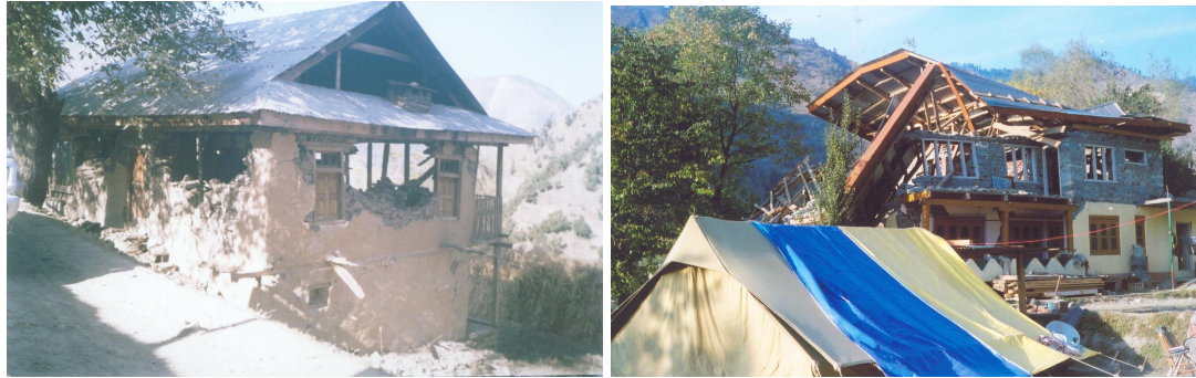
Stone masonry building on the bed rock at Kandi Concrete Building on the older alluvium (Tribuni)
