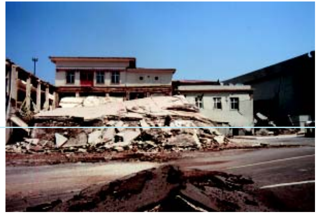
The collapsed Officer's Club at the Gölcük Naval Base. The building straddles the fault which displaced 2-3 meters. Note the faulting in the foreground.
