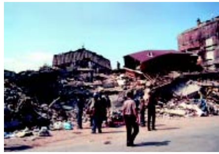
A typical, collapsed 7-story reinforced concrete commercial building in Gölcük, near the shoreline. Rescue operations in this area are in progress (middle photo). Practically undamaged shear wall building under construction in the heart of the damaged area of Gölcük (right photo).
