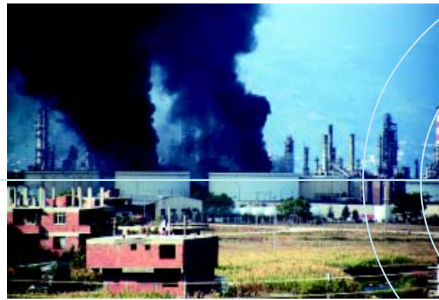
The burning Tüpras oil refinery at Korfez three days after the earthquake.
