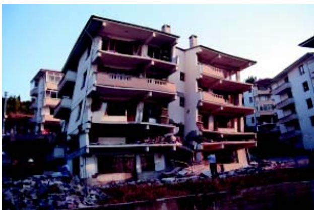
Partial collapse of and damage to new reinforced concrete apartment buildings between Gölcük and Yalova.
