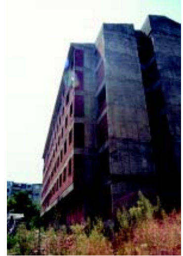
A typical, collapsed 7-story reinforced concrete commercial building in Gölcük, near the shoreline. Rescue operations in this area are in progress (middle photo). Practically undamaged shear wall building under construction in the heart of the damaged area of Gölcük (right photo).
