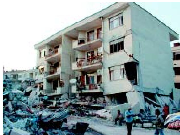
Collapsed and partially collapsed just completed 5-story buildings in Gölcük.
