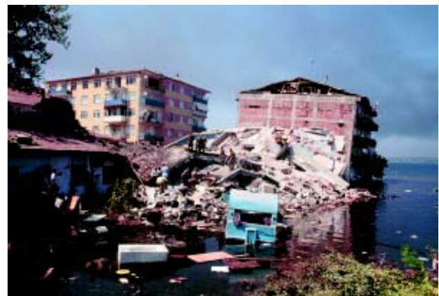
Collapsed and damaged buildings along the waterfront of Gölcük along the Sea of Marmara. The inundation is caused by a down drop of several meters along the North Anatolian fault (behind the building), combined with settlement and other ground failures.
