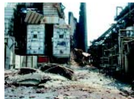
One of two collapsed cranes at the steel pipe factory in Izmit (left photo). Partial collapse of the structure caused extensive downtime at a tire manufacturing plant in Izmit (middle photo). Stack collapsed in Crude Unit, Tüpras Refinery (right photo).
