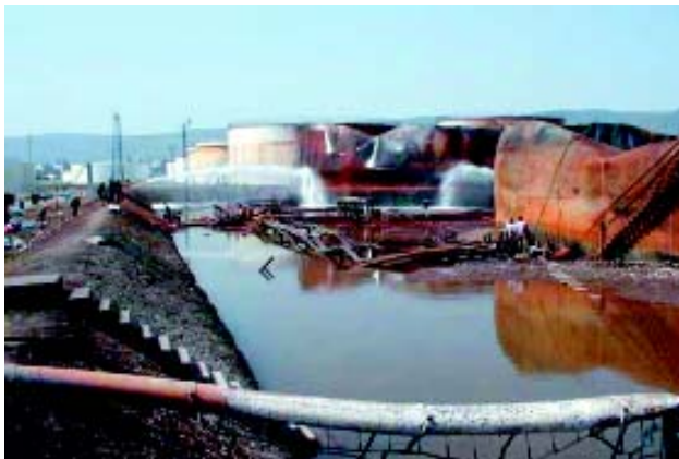
Firefighters containing tank fires at Tüpras Refinery.
