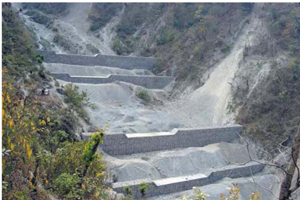
**Figure 4: Check dams built by the DWIDP in the Mugling-Narayan Ghat section to prevent debris flow**
