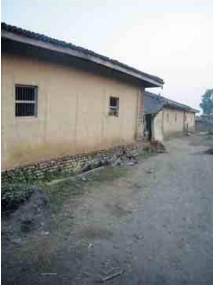
Figure 10: Mud house with brick plinths, Bhaisarawa VDC, Rautahat District
