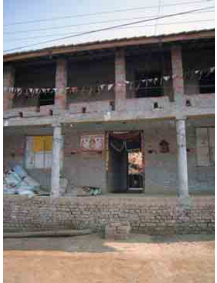
Figure 11: Elevated brick house, Katarait VDC, Dhanusha District
