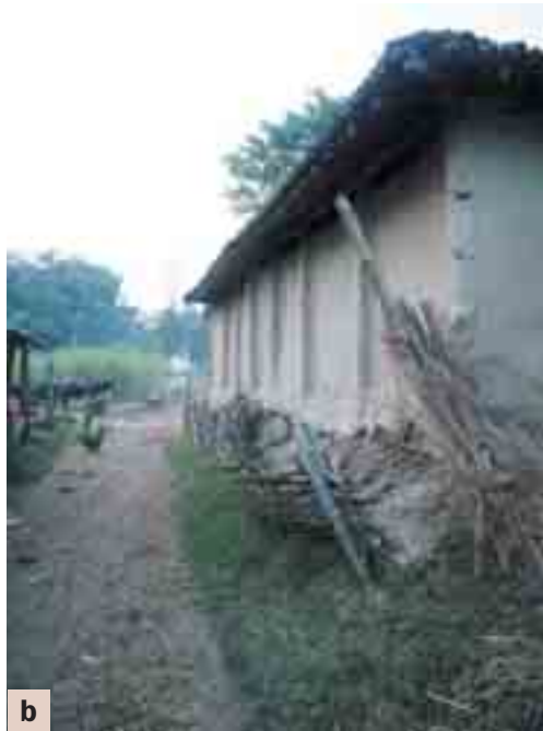
Figure 9: Strengthening and protecting walls and wall foundations: a) foundations protected with piled up mud, Katarait VDC, Dhanusha District; b) foundations protected with a bamboo fence and mud, Katarait VDC, Dhanusha District; c) wall made of bamboo, mud, and dried pulse plants supported by a wooden beam, Seurai VDC, Dhanusha District
