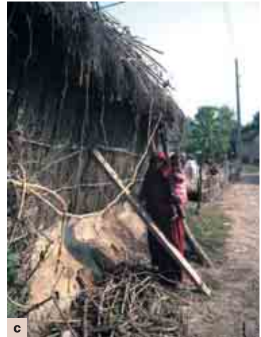
Figure 9: Strengthening and protecting walls and wall foundations: a) foundations protected with piled up mud, Katarait VDC, Dhanusha District; b) foundations protected with a bamboo fence and mud, Katarait VDC, Dhanusha District; c) wall made of bamboo, mud, and dried pulse plants supported by a wooden beam, Seurai VDC, Dhanusha District
