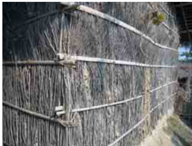
Figure 6: Walls of a local house made out of dried pulse plants, Kaitarait VDC, Dhunusha District
