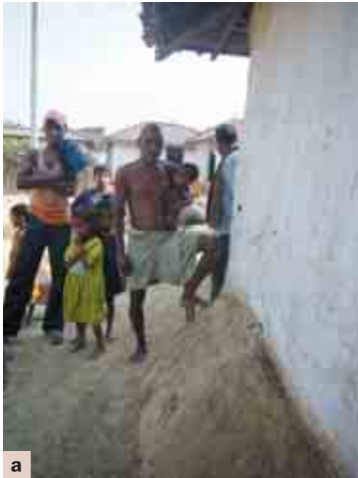
Figure 9: Strengthening and protecting walls and wall foundations: a) foundations protected with piled up mud, Katarait VDC, Dhanusha District; b) foundations protected with a bamboo fence and mud, Katarait VDC, Dhanusha District; c) wall made of bamboo, mud, and dried pulse plants supported by a wooden beam, Seurai VDC, Dhanusha District
