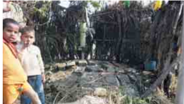
Figure 20: Water pump raised on a mud and brick platform, Katarait VDC, Dhanusha District
