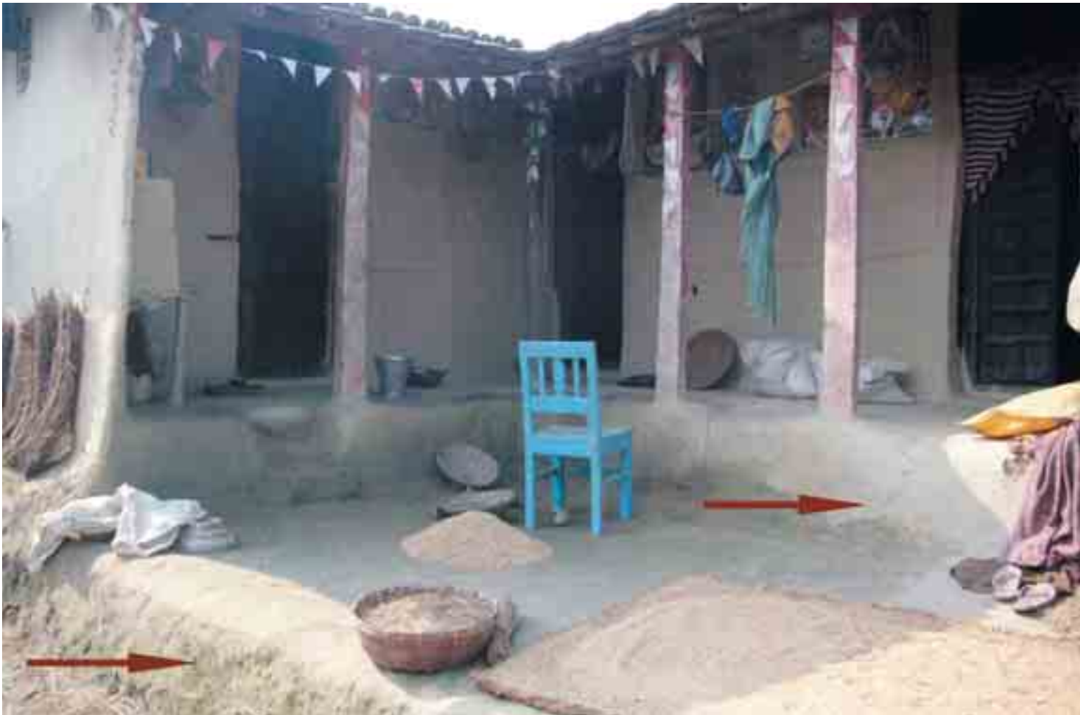
Figure 8: Mud house with two elevated mud plinths (see arrows), Katarait VDC, Dhanusha District
