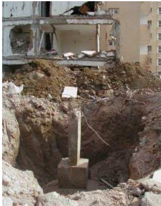
Figure 2.17. Column footings located approximately 2 m below grade at Shikhar Apartments in Ahmedabad. Photo courtesy of Tetsu Masuda.
