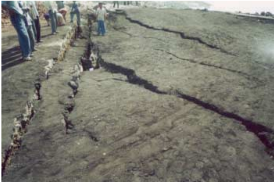
Figure 2.35. Lateral spreading due to liquefaction at the Port of Navlakhi. Photo courtesy of Svetlana Uranova.
