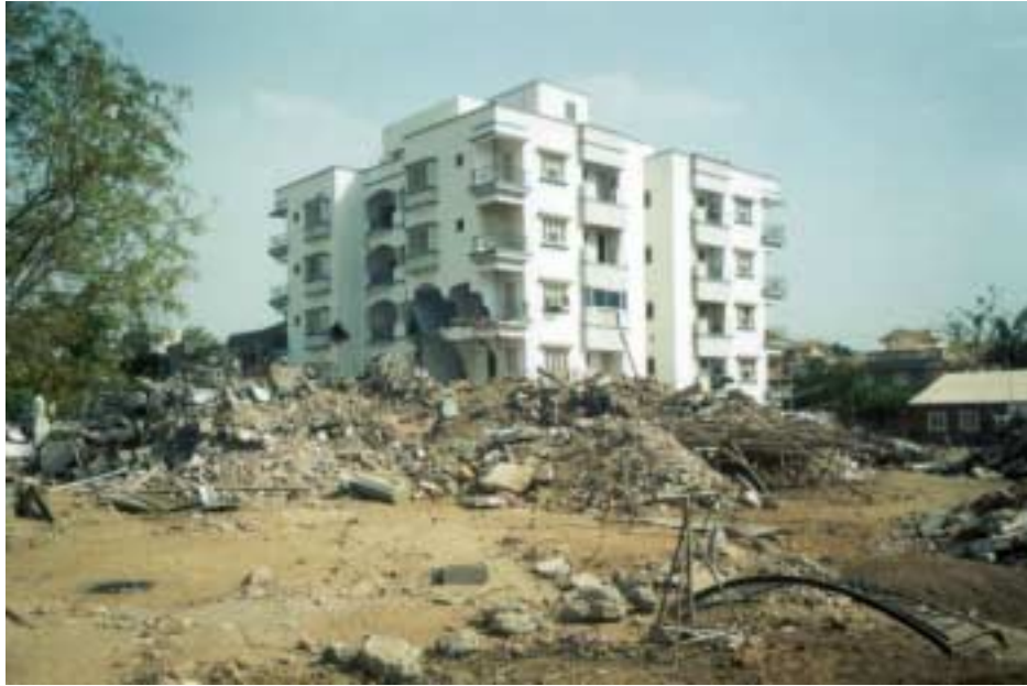
Figure 2.19. Ayodhya Apartments, Ahmedabad. Building identical to that shown collapsed as a result of soft story effects. Building in photo was significantly damaged by pounding during the collapse of the adjacent building. Photo courtesy of Svetlana Uranova.
