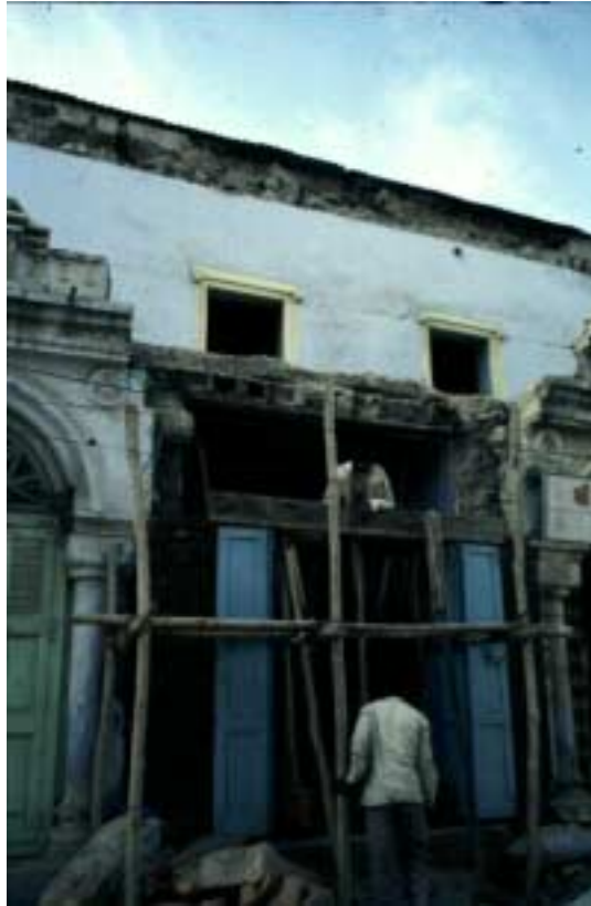
Figure 4.8. Temporary non-engineered shoring of a damaged residence, Morbi.
