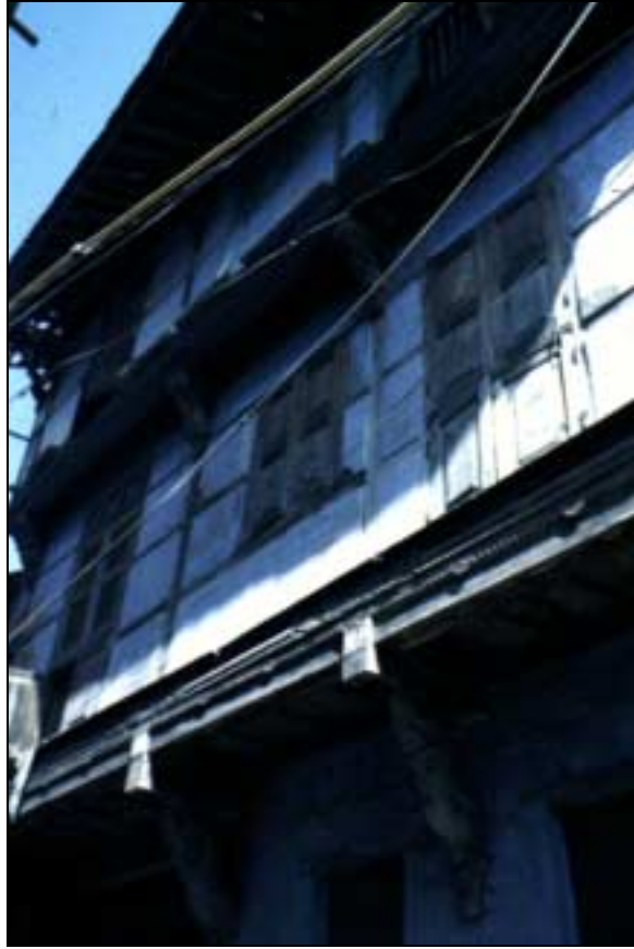
Figure 4.4. A low-rise residential structure of wooden construction, Limbdi.
