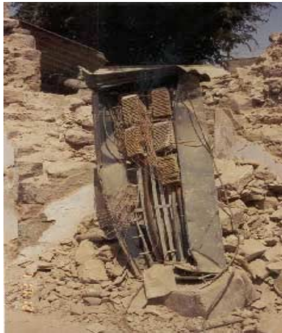
Figure 3.1. Telephone exchange, Bhachau, February 28, 2001.
