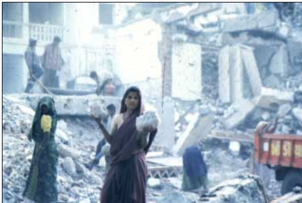
Figure 4.1. Women employed in demolition work, Ahmedabad.
