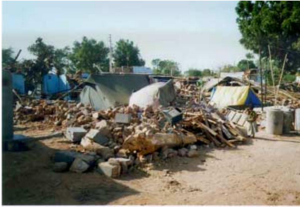
Figure 2.9. Destruction in Bhachau. Photo courtesy of Ahmad Naderzadeh.
