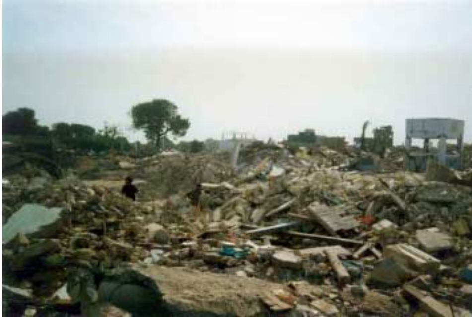
Figure 2.11. Destruction in Bhuj. Photo courtesy of Ahmad Naderzadeh.
