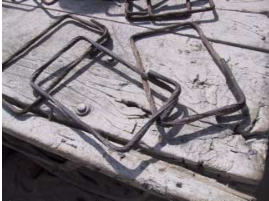
Figure 2.25. Evidence at a new construction site in Ahmedabad that 90° hooks instead of 135° hooks are still used for column ties. Photo courtesy of Weimin Dong.
