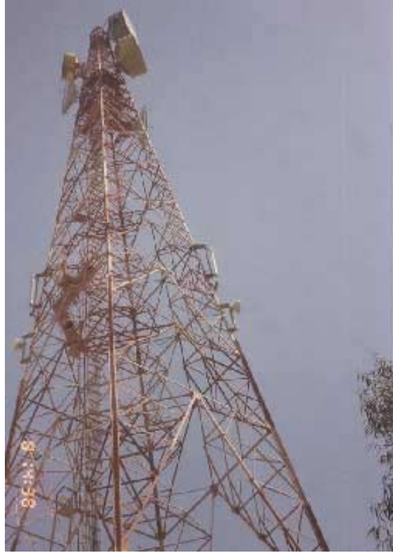
Figure 3.6. Telecommunications tower, Gandhidham, March 2, 2001.
