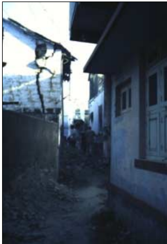
Figure 4.7. Rubble still exists one month after the earthquake, Morbi.
