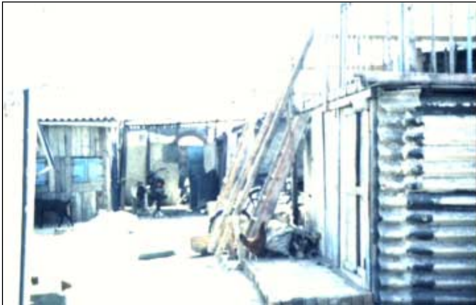
Figure 4.3. Typical housing constructed of tin plates, Navlakhi.
