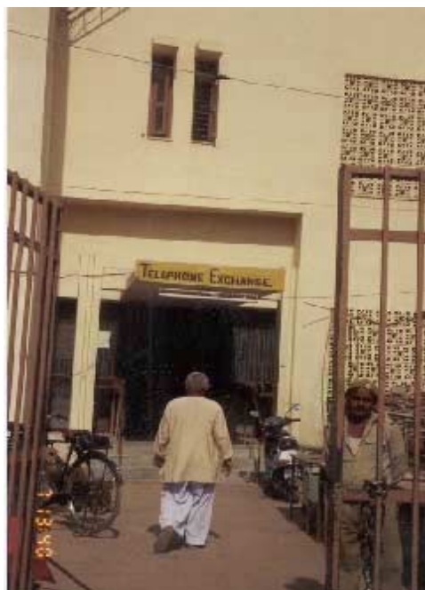
Figure 3.5. Telephone Exchange, Anjar, March 1, 2001.
