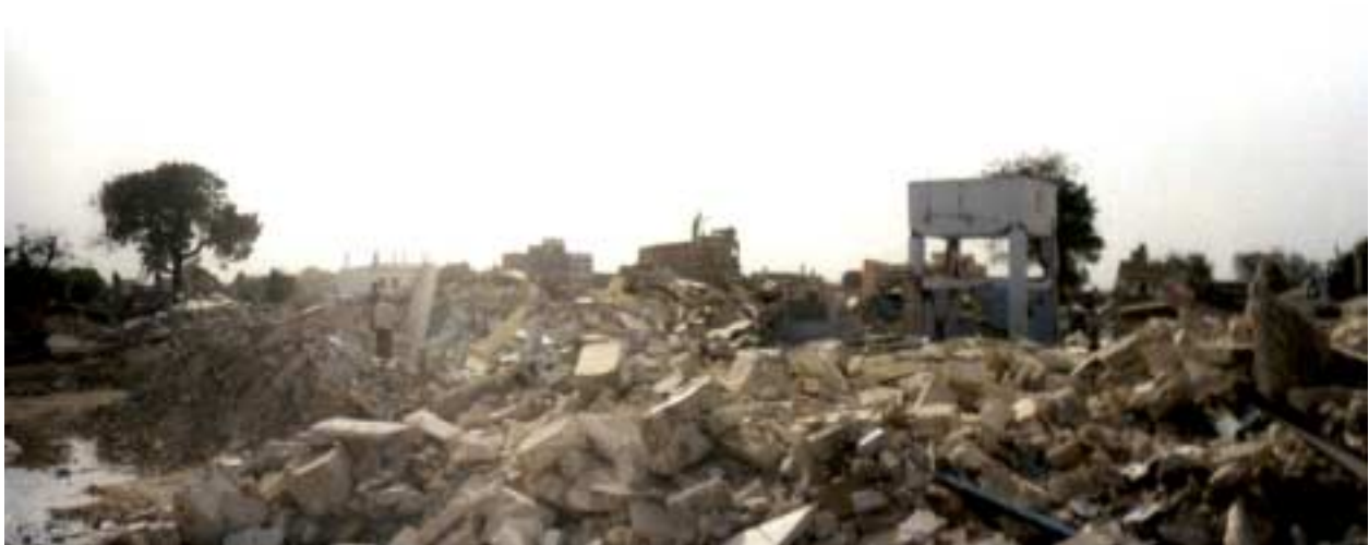
Figure 2.4. Destruction of masonry structures in the old section of Anjar. Photos courtesy of Charles Menun.
