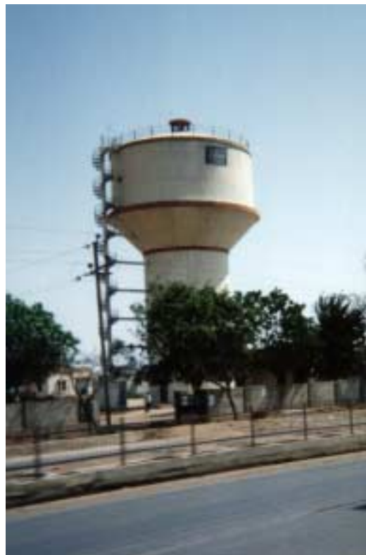
Figure 2.44. Government-designed elevated water tank near Gandhidham. No apparent damage. Photo courtesy of Charles Menun.
