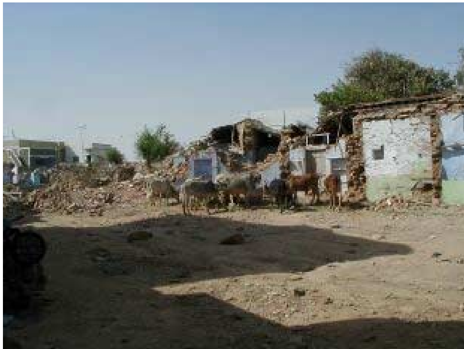
Figure 2.10. Most stone houses in the old town of Bhuj collapsed. Photo courtesy of Tetsu Masuda.
