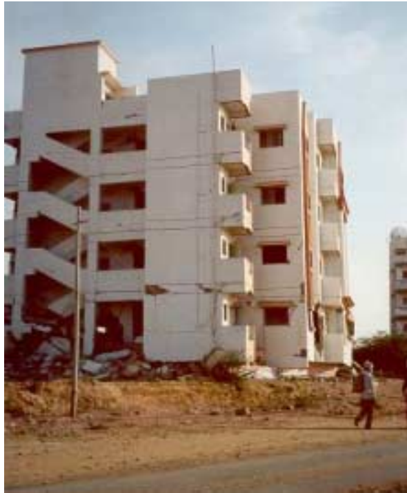
Figure 2.21. Soft story collapse of a five-story apartment building in Bhuj. Photo courtesy of Amod Dixit.
