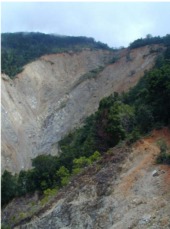
Figure 2. View to the northeast of the upper part of El Zompopera landslide. The collapse of unstable blocks in the upper part of the landslide destroyed a road at the crest of the ridge. Many unstable blocks remain in the upper part of the slide and a catastrophic collapse of those blocks could potentially dam the Río La Palma at the bottom of the valley. A catastrophic failure of a landslide dam could cause flooding and damage in the downstream town of La Palma.
