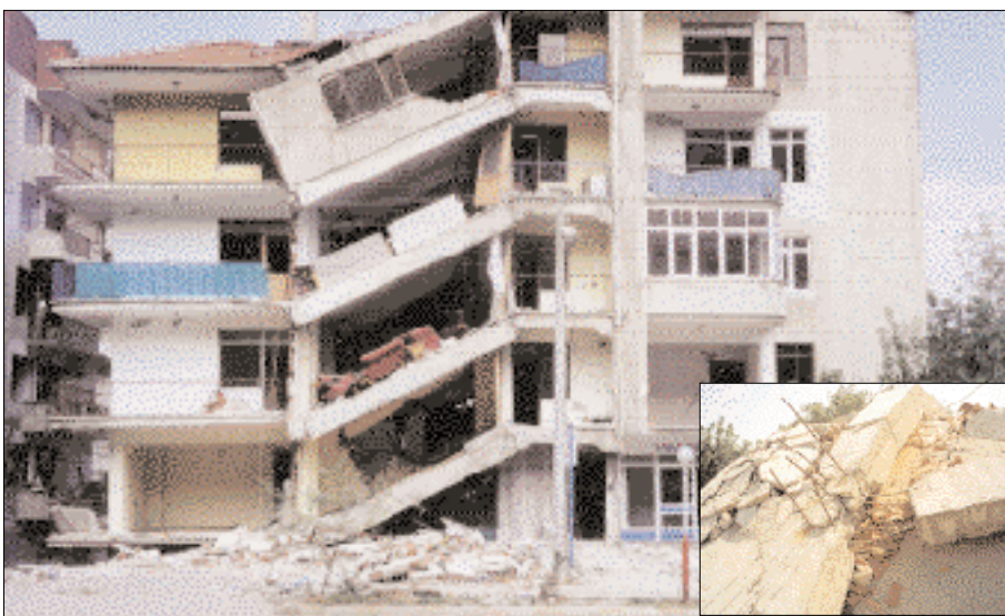
Commonly seen throughout the epicentral region, a portion of this reinforced concrete building's first floor was partially destroyed. As shown in the inset, columns generally lacked an adequate amount of steel reinforcement.
