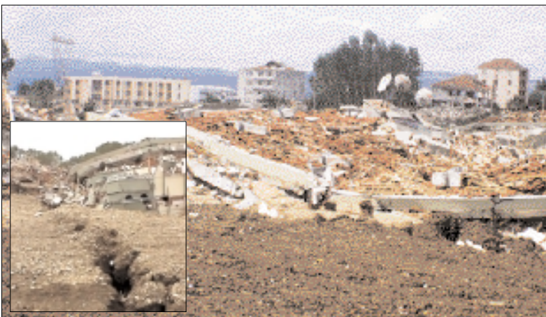
The fault ruptured through this recently built but unoccupied 180-unit vacation development near Kular, completely destroying 7 of 8 buildings. The remaining building and all surrounding structures were also heavily damaged.
