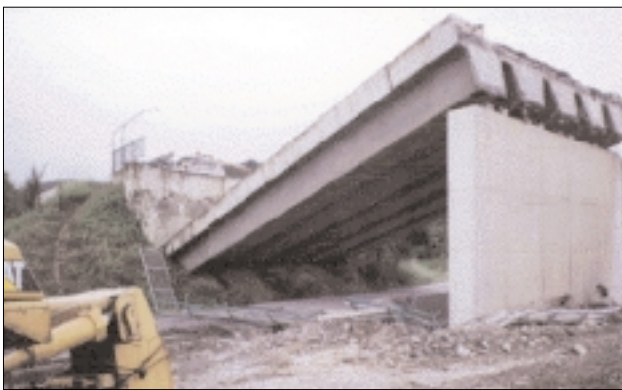
The fault rupture severed this bridge from its approach, along the Istanbul-Ankara motorway.
