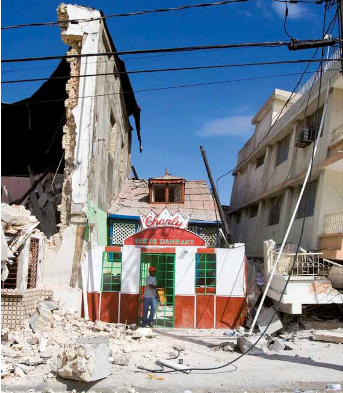
Port-au-Prince, Haiti, 2010: It is not the earthquakes that kill people, but the buildings collapsing on them.
