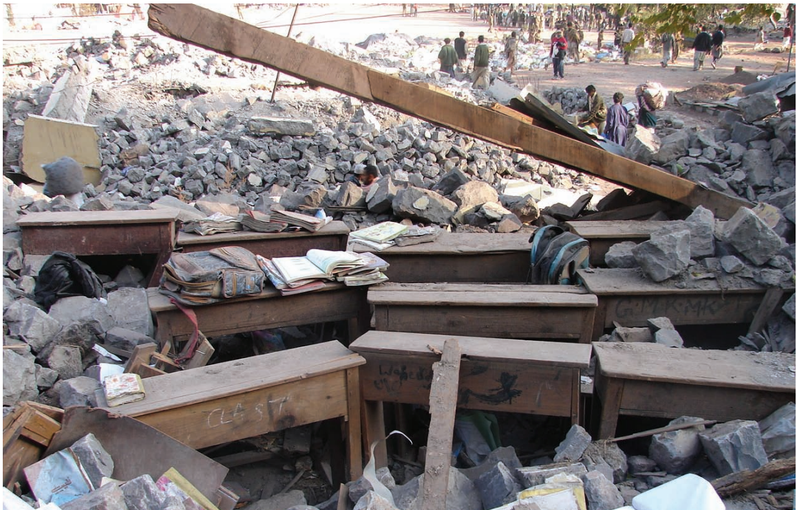
67% of schools and colleges in AJK and NWFP were destroyed/damaged by the earthquake, and 18,000 students killed.
