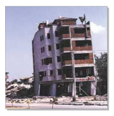
**Figure 43.** Near collapse of building in Adapazari as the result of formation of column hinges in the first story. *Photograph by National Institute of Standards and Technology*.
