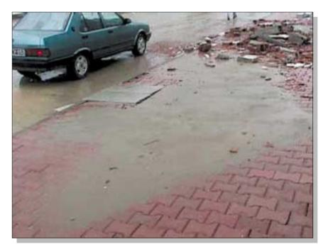
**Figure. 36.** Sand boil on sidewalk in Adapazari. Sand ejected from underground when sandy soils beneath the ground-water table liquefied during the earthquake. *Photograph by Mehmet Çelebi.*
