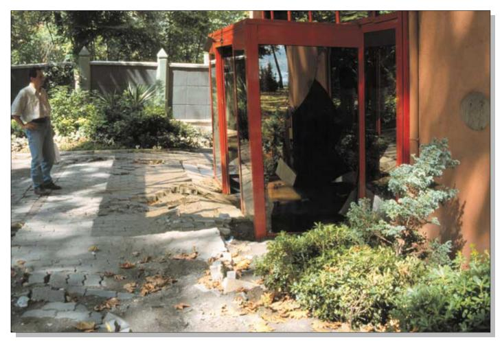
Figure 38. Sunken entryway into Sapanca Hotel created when building sank into liquefied soil. Photograph by Thomas L. Holzer.
