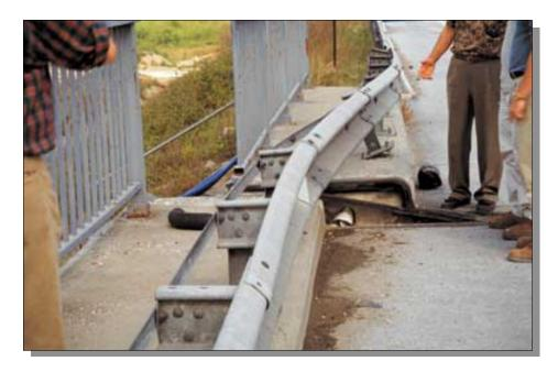
Figure 51. Ground shaking caused the westbound span of the Sakarya River bridge to displace 50 cm relative to the east abutment. This was the largest permanent displacement caused by shaking at any bridge. Photograph by Selcuk Toprak.
