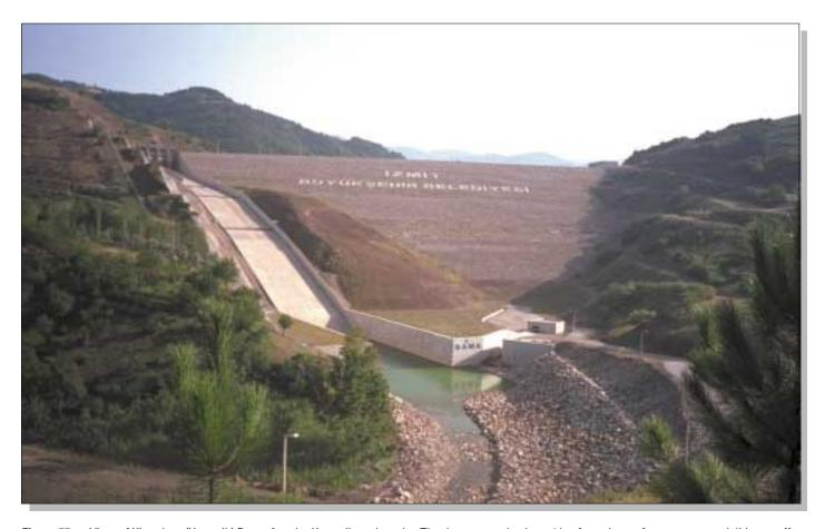
**Figure 55.** View of Kirazdere (Yuvacik) Dam after the Kocaeli earthquake. The dam was only about 4 km from the surface rupture and did not suffer damage. *Photograph by Richard S. Olsen.*
