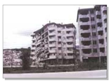
**Figure 42.** Partial collapse of building near Izmit as the result of shear failure of intermediate columns. Note various stages of damage despite apparently similar construction. *Photograph by National Institute of Standards and Technology.*
