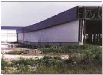
**Figure 45.** Industrial building damaged by near-fault ground movements east of Gölcük. Building is on downthrown block of normal fault and near a major change of strike in the surface fault scarp. *Photograph by National Institute of Standards and Technology.*
