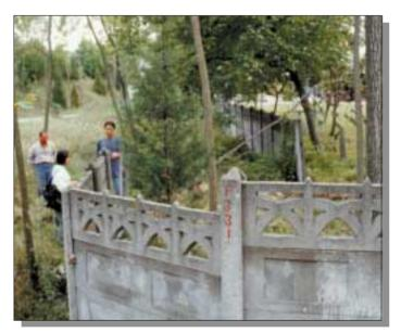
**Figure 18.** Offset wall near Arifiye. The right-lateral displacement is 4.58 m. *Photograph by Heidi Stenner.*
