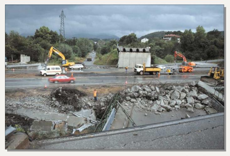
**Figure 53.** The Arifiye overpass collapsed because the surface fault rupture passed directly through its north abutment (foreground). Ten riders of a bus were killed when the bus collided with the collapsed overpass. *Photograph by Thomas L. Holzer.*
