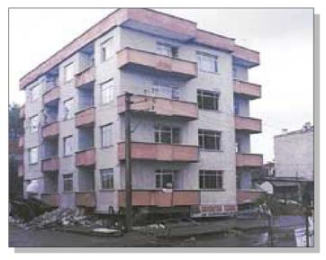
**Figure 41.** Partial building collapse in Yalova as the result of shear failure of first story columns. *Photograph by National Institute of Standards and Technology.*
