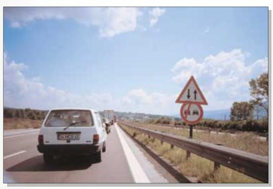
**Figure 48.** Following the earthquake, road surface repairs forced alternative use of the eastbound and westbound lanes of the Trans European Motorway as a two-way highway with greatly reduced speeds from Izmit to about 50 km east of Izmit. *Photograph by Thomas L. Holzer.*
