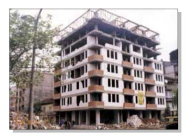
**Figure 40.** Building in Izmit under construction using reinforced concrete frame construction. Note absence of shear walls. *Photograph by National Institute of Standards and Technology.*
