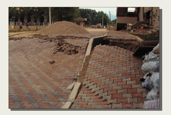
Figure 10. Tectonic scarp along the normal fault in Gölcük in a cobblestone pavement with both vertical (~1 m) and horizontal (~0.3 m) components of offset. *Photograph by Robert Langridge*.
