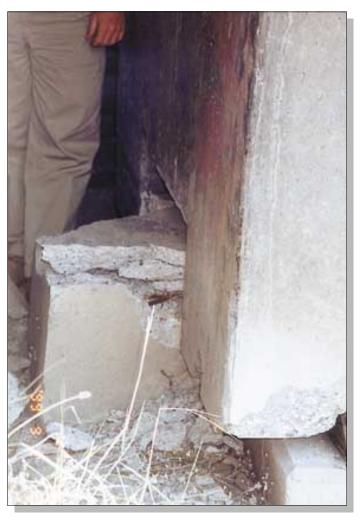
**Figure 50.** Failure of shear keys was common at bridges of the Trans European Motorway. Shear keys at the end of girders prevent transverse and longitudinal seismic movements. *Photograph by Selcuk Toprak*.
