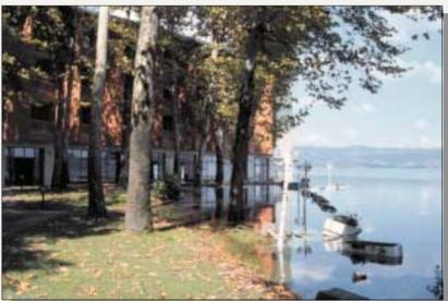
**Figure 37.** Submergence of shoreline at Lake Sapanca and settlement of Sapanca Hotel. "Moat" adjacent to wall indicates the hotel has sunk into the ground because of liquefaction of underlying sandy soil. *Photographs by Thomas L. Holzer.*
