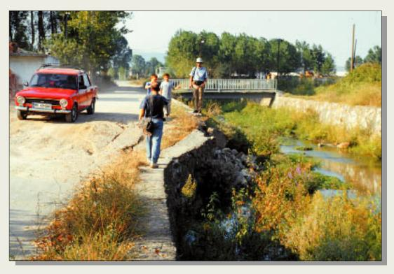
Figure 14. Offset canal near lzmit. Strike-slip displacement across the whole zone here was more than 2.5 m and included a vertical component (middle left). Photograph by Heidi Stenner.
