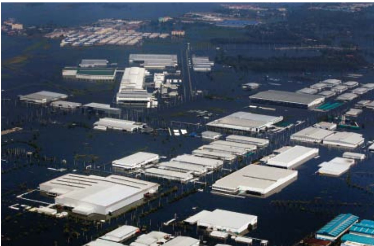
The Rojana industrial park near Ayutthaya was completely flooded and production was at a standstill for weeks on end.
