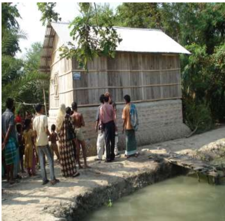
Fortified plinth in Bangladesh
