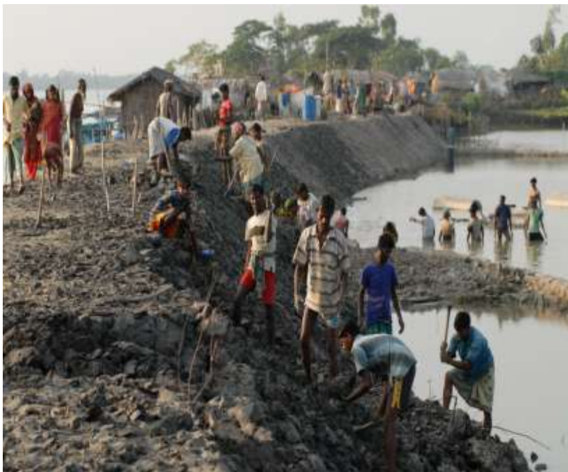
Construction of dikes in India (pic. Th. Hirsch)
