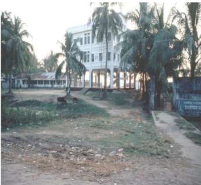
Cyclone shelter in Bangladesh
