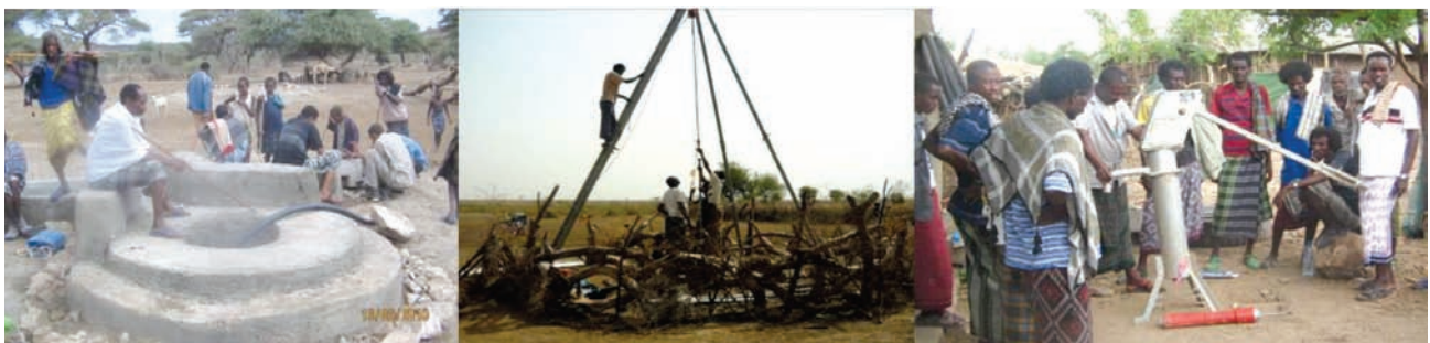
Traditional wells being upgraded
