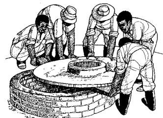
Set the cured well cover in place.
