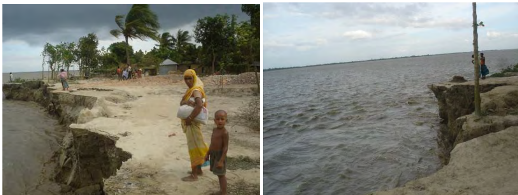
Figure 3-20. Figure. Already started riverbank erosion in many locations of the pilot area.
