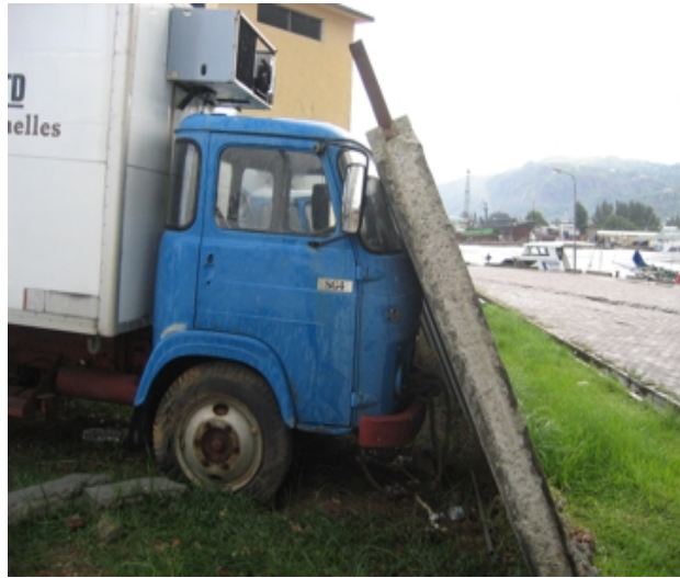
Fig. 11: Concrete wall toppled by the force of the tsunami, inner harbour, Victoria. Photo: LEJ (GSC), 25 Jan 2005.
