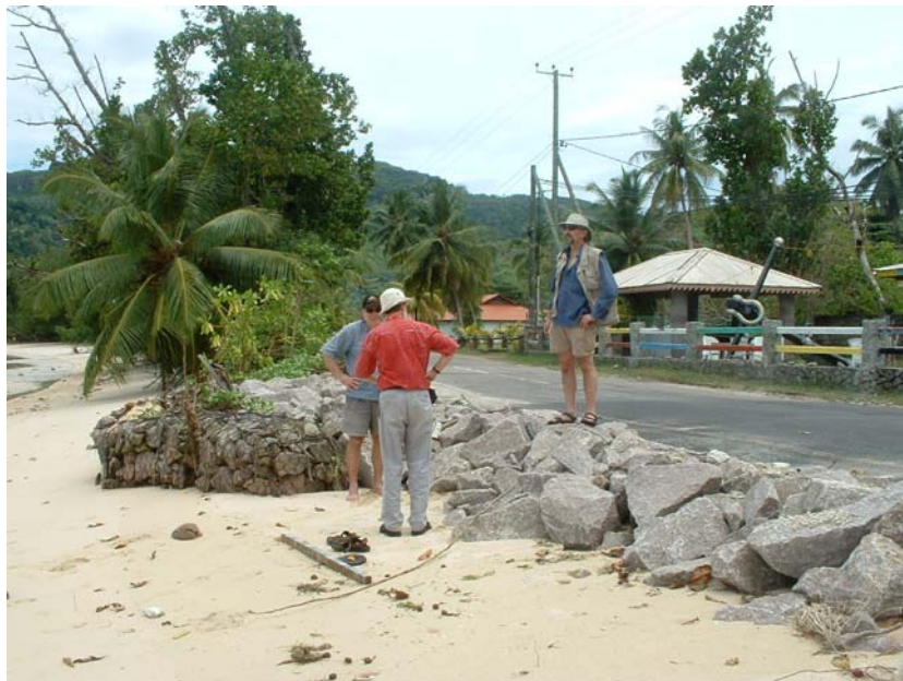
Fig. 43: The seafront at Anchor Café. Note the low boulder rip rap, the road, and the café beyond. Prior to the tsunami, there was enough land on the seaward side of the road for a kayak shed. Photo: JS (GSC), 26 Jan 2005.
