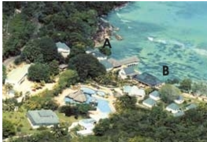
Fig. 61: A- La Reserve Hotel. All of the buildings between points A and B will have to be demolished because of structural failure due to undermining of their foundations by the draining tsunami flood. The pier restaurant is midway between the two letters. North is toward the right. Virtually the entire property was inundated by the tsunami. Photo from http://www.mauritius-seychelles.com/la-reserve-hotel-seychelles.html .
