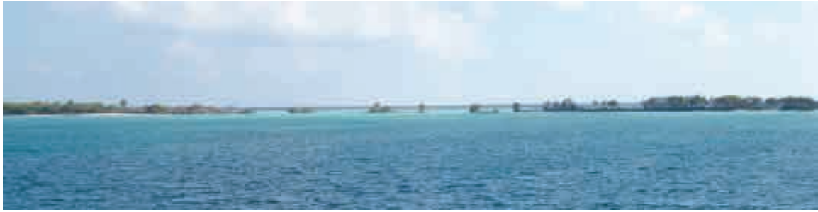
FIGURE 4.19: The breach in Kalhufahalafushi.
