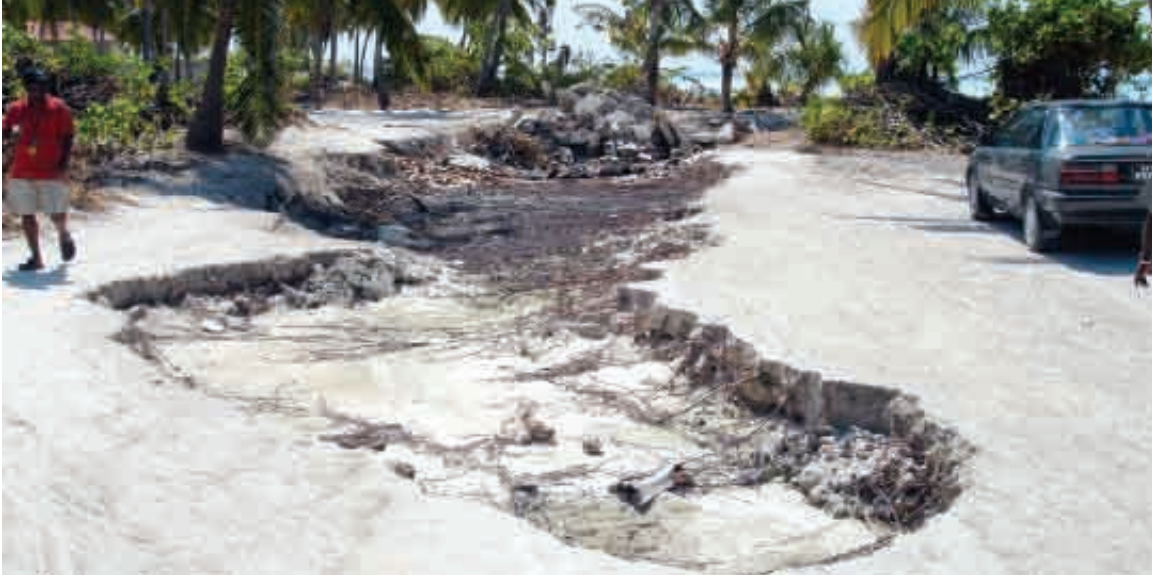
FIGURE 4.10: Gully erosion by return flow at the northern end of Gan.
