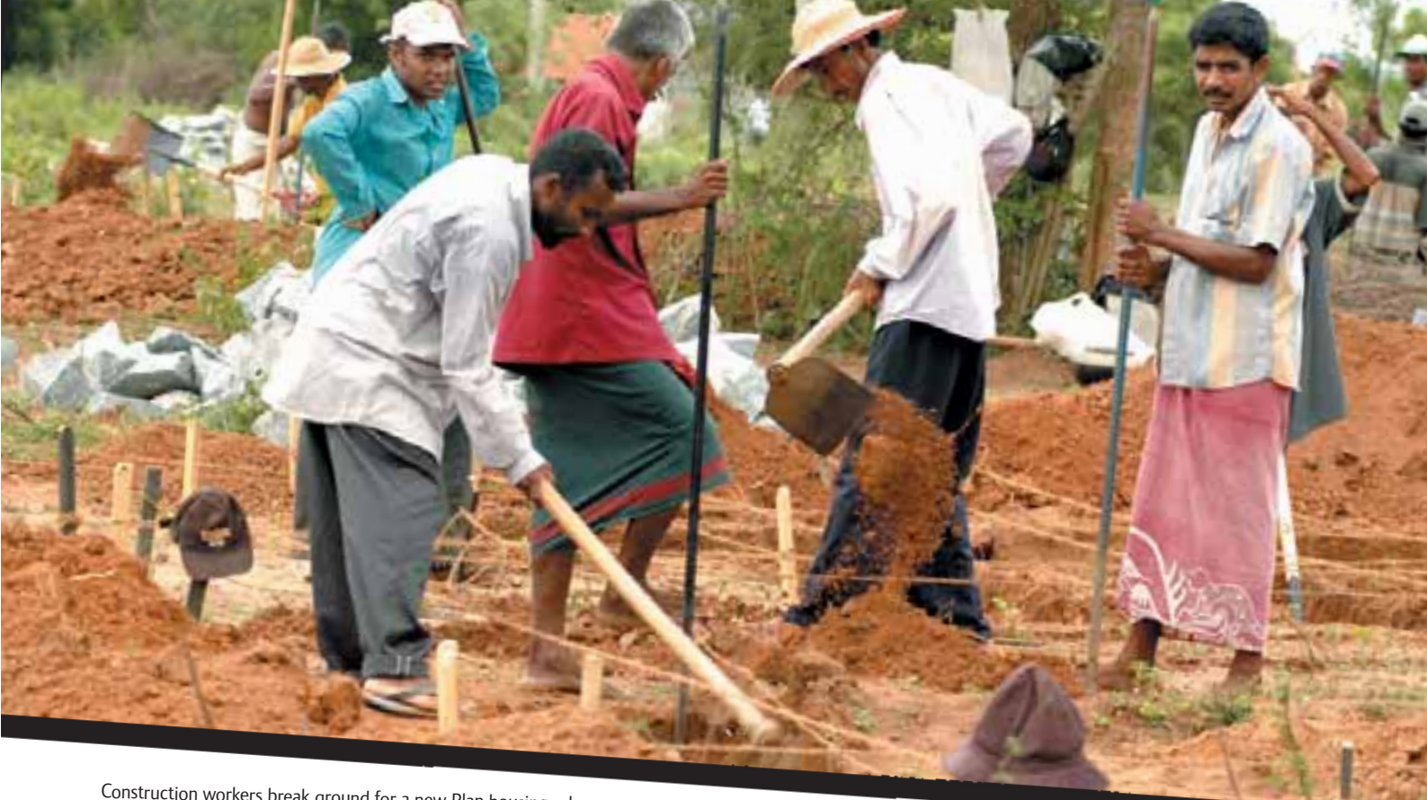
Construction workers break ground for a new Plan housing scheme in Tangalle Division.
