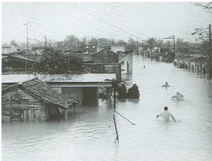
Floods in Cuba in the aftermath of Hurricane Albert, 1982
