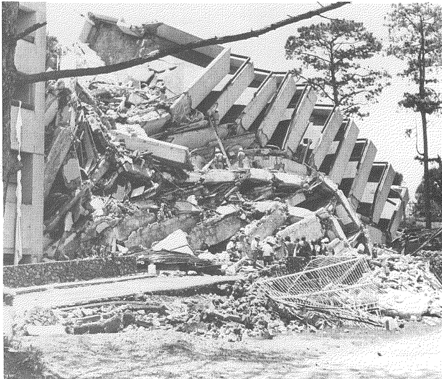
A hotel in Baguio City, Philippines, collapsed in the earthquake of July 1990, killing hundreds.
