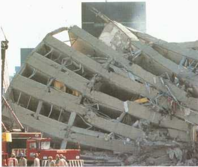
Collapsed building after Mexico City earthquake, 1985.
