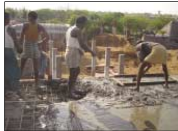
Leveling of roof concrete
