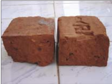
Large aggregates causing splitting and weakening of the brick
