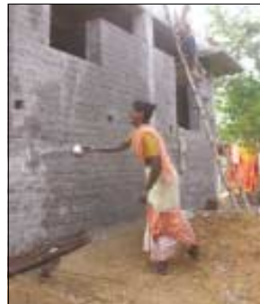
Curing of the brickwork
