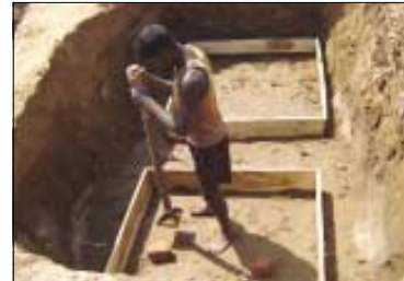
Ramming the foundation pit
