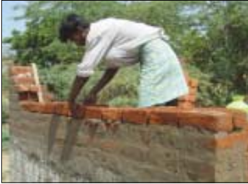
Using string to ensure the horizontality of brickwork
