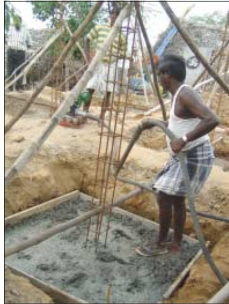
Vibrator is used for compacting the concrete
