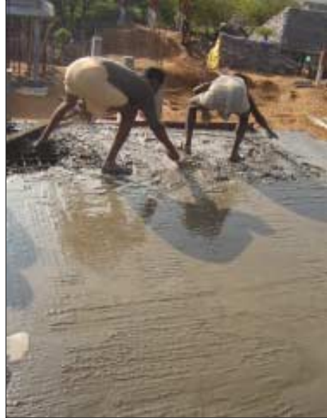
Finishing the roof slab by plastering
