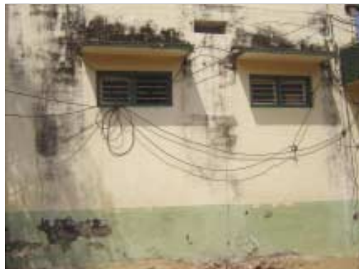
Wall below sunshade is in good condition
