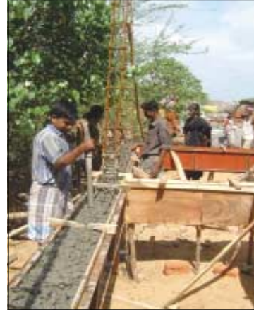
Compacting concrete using the vibrator
