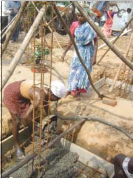
Pouring concrete at lower height
