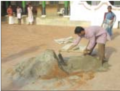
Dry mixing of cement and sand
