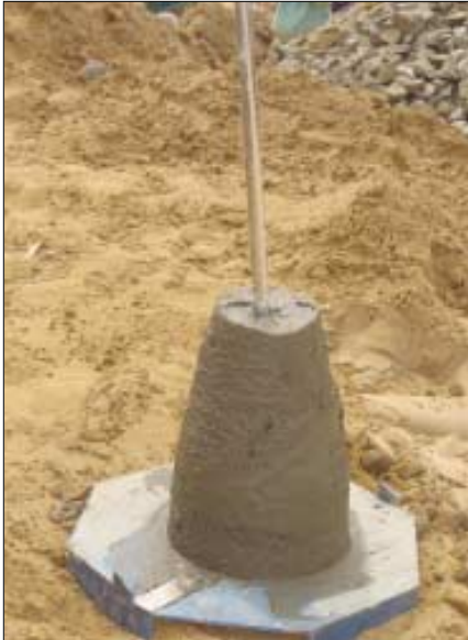
Slump cone test
