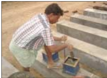
Concrete cubes cast at the site for testing the compressive strength
