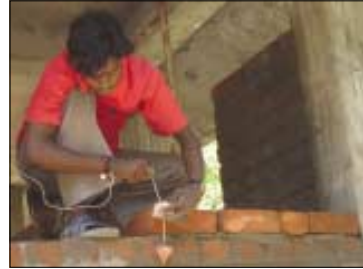
Checking the plumbness of the wall at regular intervals
