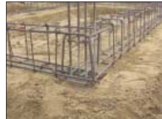
Beam main bar bent at the end to have column to beam connection
