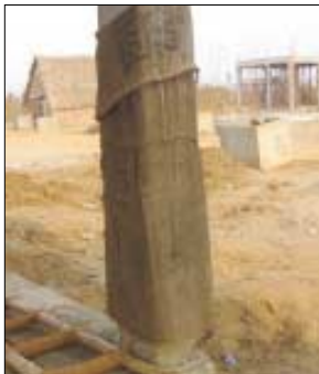
Wet Gunny bags wrapped to keep the concrete wet
