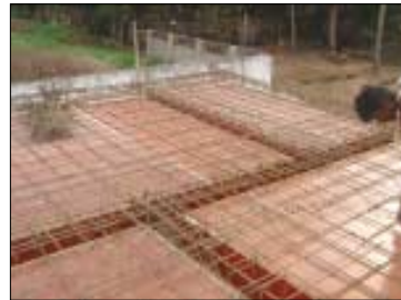
Roof slab formwork with reinforcement
