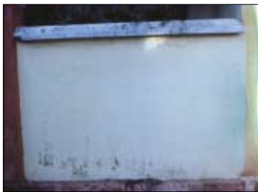
Coping to protect the brickwork below
