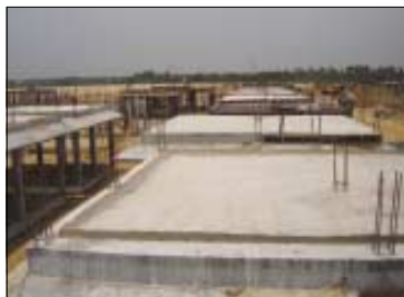
For roof slabs, water should be stagnated by constructing small bunds
