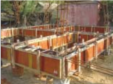
Grade beam formwork
