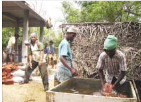
Soaking of bricks
