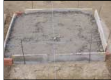
Centre line marking to fix the mat and column reinforcement
