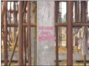
Column concrete with good finishing
