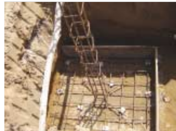
Cover block for footing
