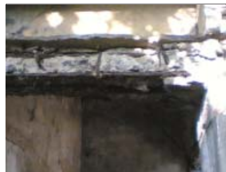
Damaged Roof Beam
