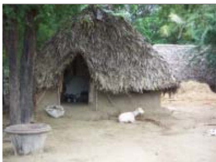
Low Mud Wall and Palm Thatch Roof
