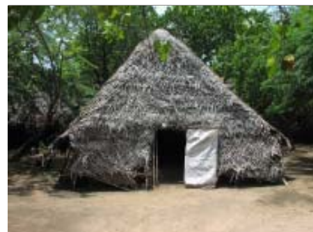
Coconut Thatch as Walling and Roofing Material
