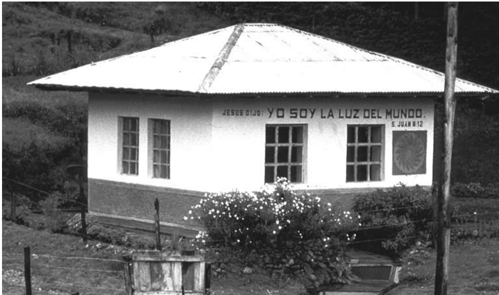
Micro Hydro Power House. Photo: © Practical Action/Colin Palmer
