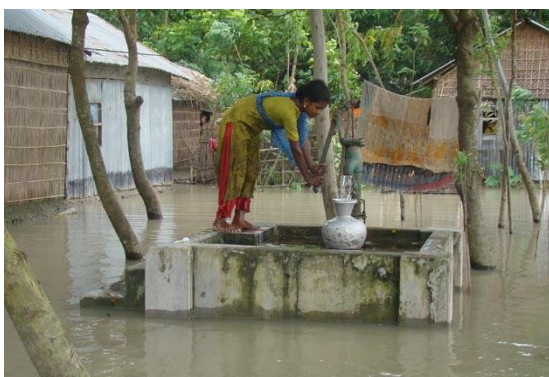
A hand pump raised above flood waters
