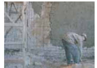
School retrofitting work Tashkent, Uzbekistan
