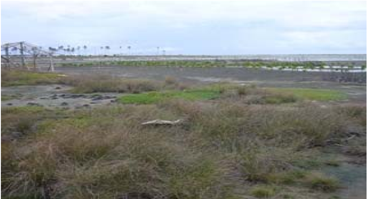
Figure 2. CRC housing construction site- some portion is very close to ocean and is swampy
