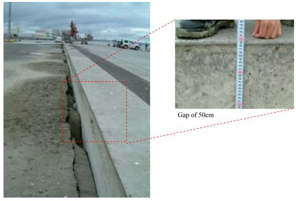
Photo A3.e - Damage to port facility.
