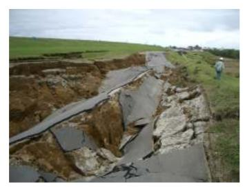
Photo A3.b - Embankment damage due to slope failure (Tokachi river).
