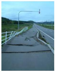
Photo A3.d – Bank failure
