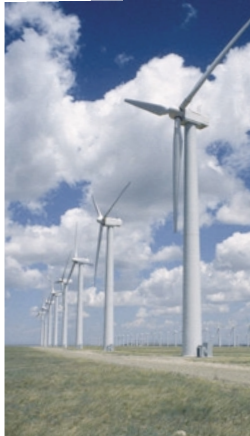
Photo: Eugene Water and Electric Board
