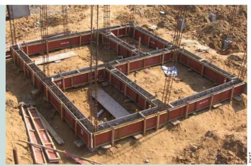
The ground under the building needs to be strong enough to support the building, even if it is flooded or exposed to earthquakes. A proper assessment of the underground and removal of overlying earth of poor quality is essential in all cases.
