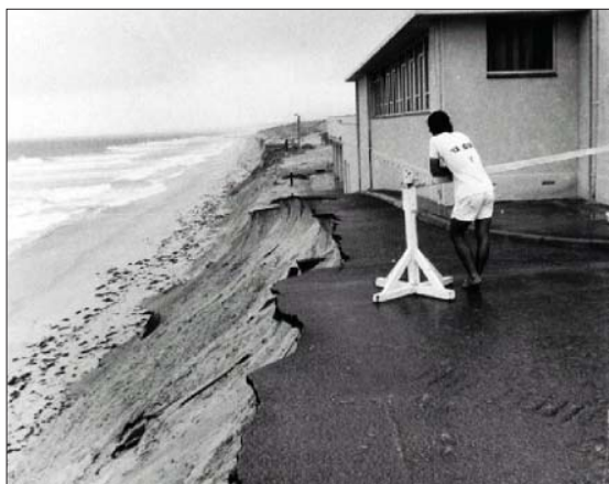
Figure 9: Coastal erosion on Perth's beaches as a result of Tropical Cyclone Alby in 1978 (Courtesy of The West Australian).
