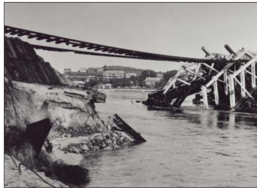
Figure 5: Fremantle Railway Bridge destroyed by the July 1926 floods (Courtesy of the Batty Library 54902P).
