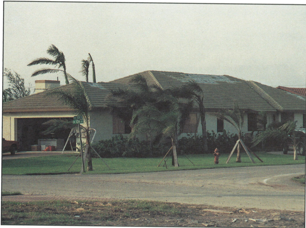
FIGURE 38. Hip roof.
