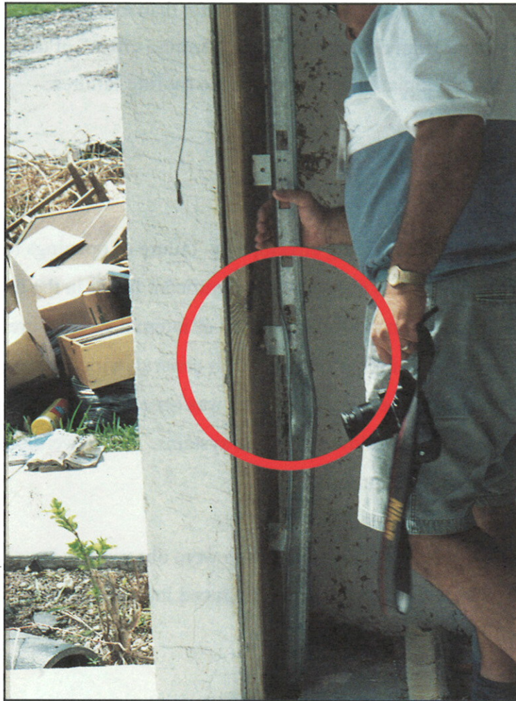
FIGURE 25. Garage door failure. Rotation of track, and pullout of brackets at wall support.
