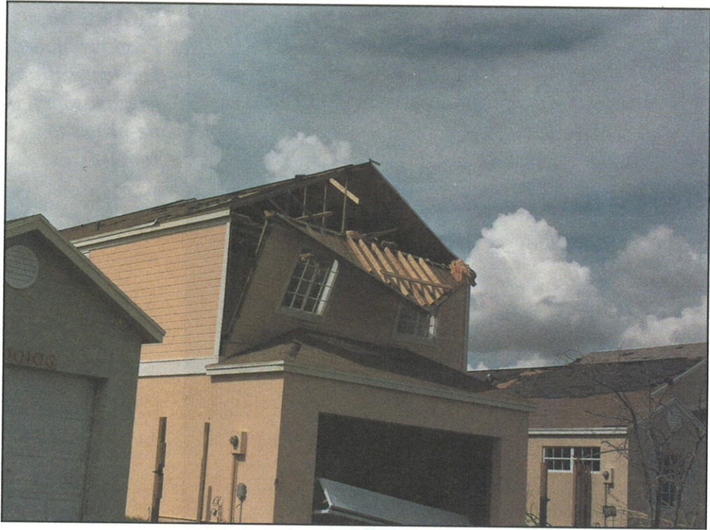
FIGURE 58. End wall failure. Example of lack of load transfer capacity after separation.
