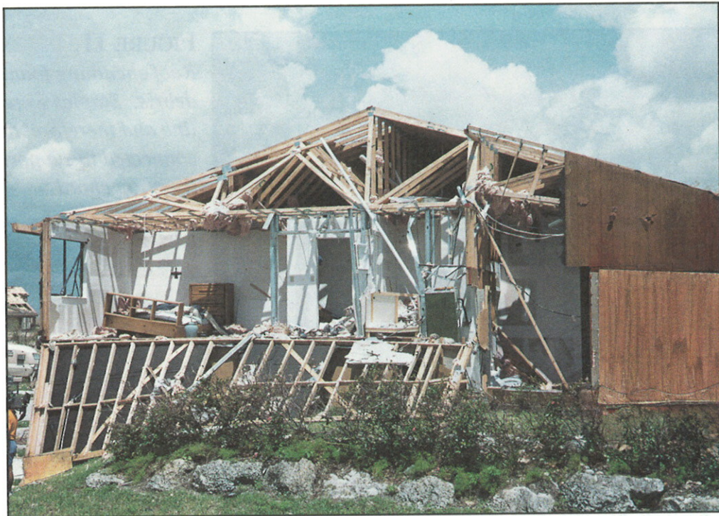
FIGURE 12. End wall failure of typical first floor masonry/second floor wood-frame building. Truss bridging and lateral bracing, and adequately installed roof sheathing, would have greatly reduced the likelihood of such a failure.
