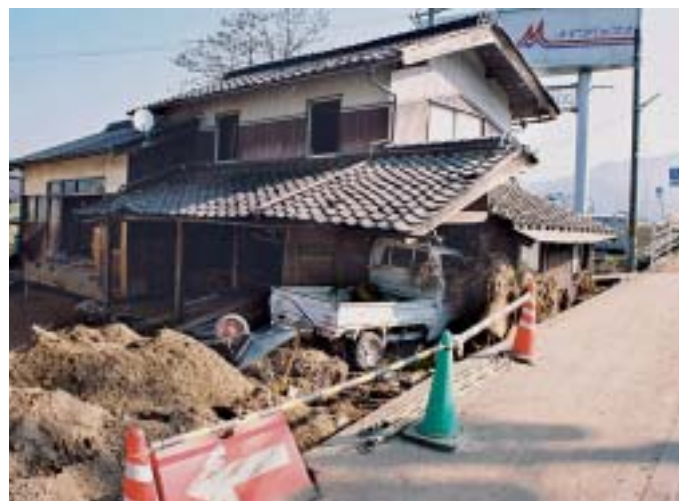
Typhoon Tokage sped over Japan with wind speeds of up to 200 km/h. Buildings and infrastructure were severely damaged particularly in the region of Okinawa.
