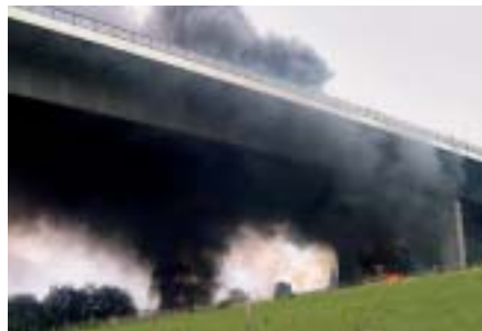
26 August, Germany, Gummersbach Accident on a motorway bridge
