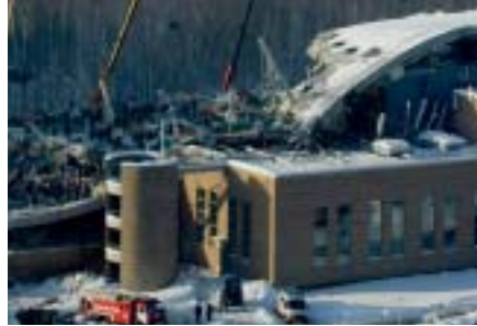
14 February, Russia, Moscow Roof collapse at an indoor swimming pool
