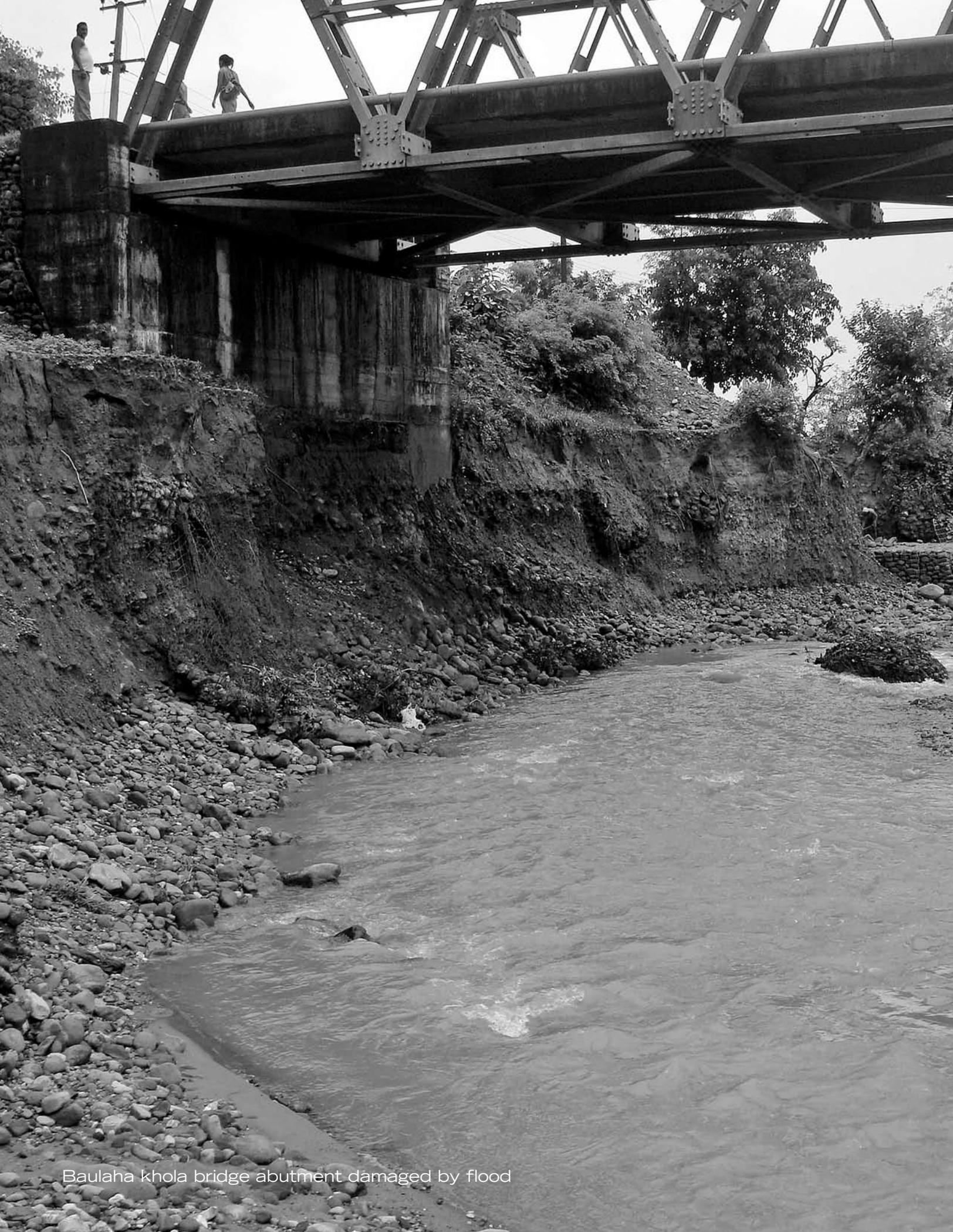
Baulaha khola bridge abutment damaged by flood
