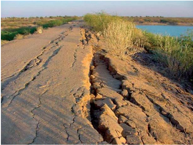
Above left to right: Different types of damage of embankment dams caused by the magnitude 7.5 Bhuj earthquake in Gujarat province, India, January 26, 2001. Mainly small dams for irrigation and water supply were damaged. Right: Damage of reinforced concrete buildings on top of intake towers of the Zipingpu reservoir, May 12, 2008 Wenchuan earthquake
