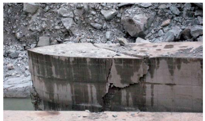
Above left to right: Different types of damage of embankment dams caused by the magnitude 7.5 Bhuj earthquake in Gujarat province, India, January 26, 2001. Mainly small dams for irrigation and water supply were damaged. Right: Damage of reinforced concrete buildings on top of intake towers of the Zipingpu reservoir, May 12, 2008 Wenchuan earthquake
