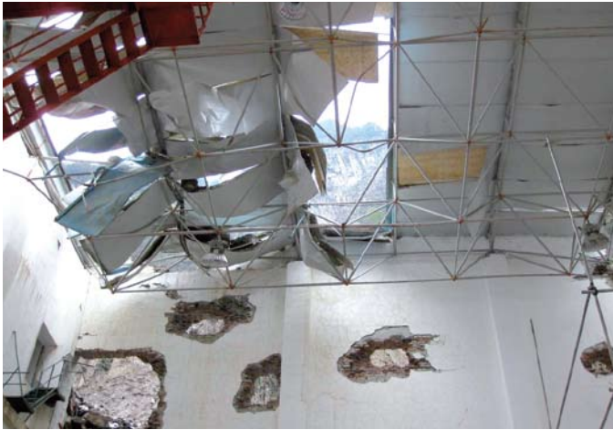
Above left: Damage of the Shapei powerhouse caused by rockfall during the May 12, 2008 Wenchuan earthquake; Above right: Sheared off pier of Futan weir at the Minjiang river due to the impact of large rocks, May 12, 2008 Wenchuan earthquake
