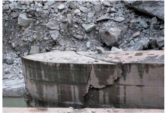
Above left: Damage of the Shapei powerhouse caused by rockfall during the May 12, 2008 Wenchuan earthquake; Above right: Sheared off pier of Futan weir at the Minjiang river due to the impact of large rocks, May 12, 2008 Wenchuan earthquake
