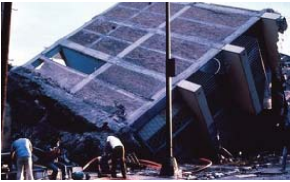
Figure 2. Liquefaction effect after Mexico Earthquake in 1985
