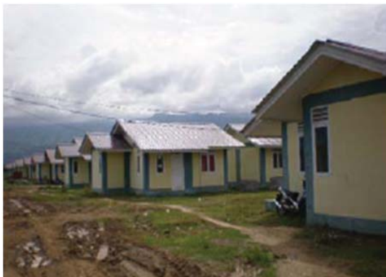
Figure 1. Lack of need assessment caused many houses that were ready were not yet occupied.
