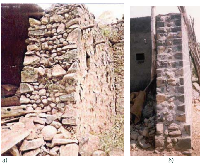
Figure 1. Stone masonry construction in Maharashtra, India: a) traditional construction (before the earthquake), and b) improved construction practice.
