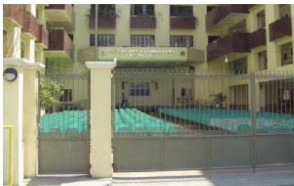
Figure 4. Barangay Rizal Elementary School, © EMI
