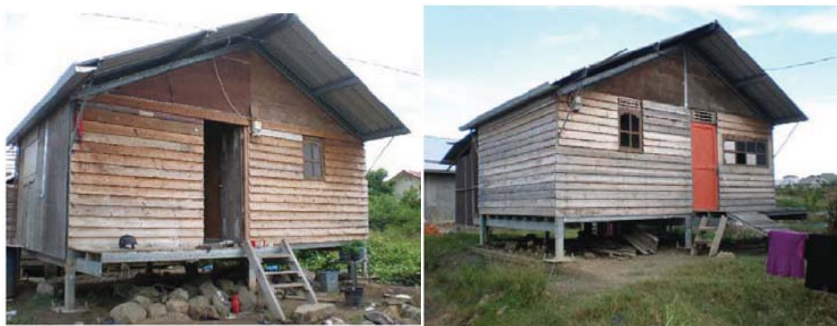
Figure 2. “Temporary/ transition” houses become permanent. Pictures were taken at the end of November 2008.
