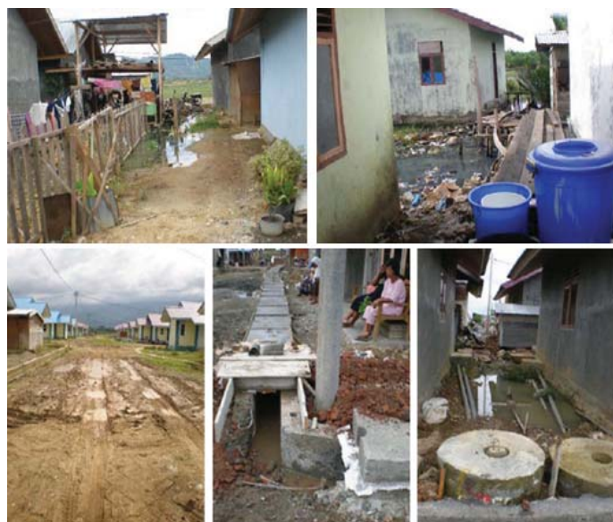
Figure 3. Site engineering construction activity did not run parallel with the site layout planning. All pictures were taken at the end of November 2008.
