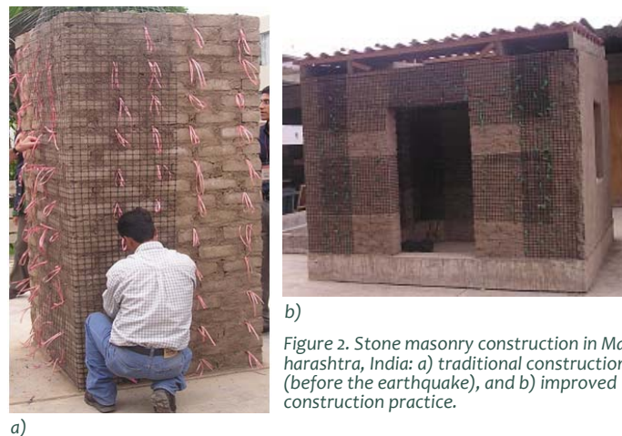
Figure 1. Stone masonry construction in Maharashtra, India: a) traditional construction (before the earthquake), and b) improved construction practice.
