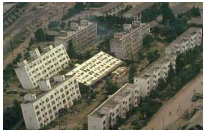
Figure 1. Collapse of building after Niigata earthquake in 1964
