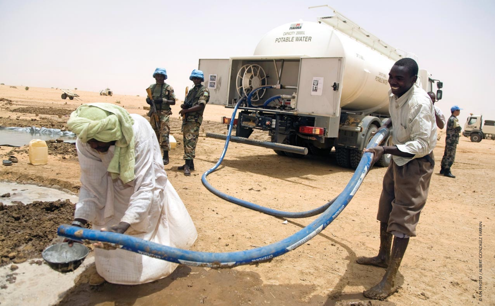
The Disarmament, Demobilization and Reintegration Section of the African Union-United Nations Hybrid Operation in Darfur (UNAMID) delivers water to construct a school that will house 30 former child soldiers, in Tora village, North Darfur.
