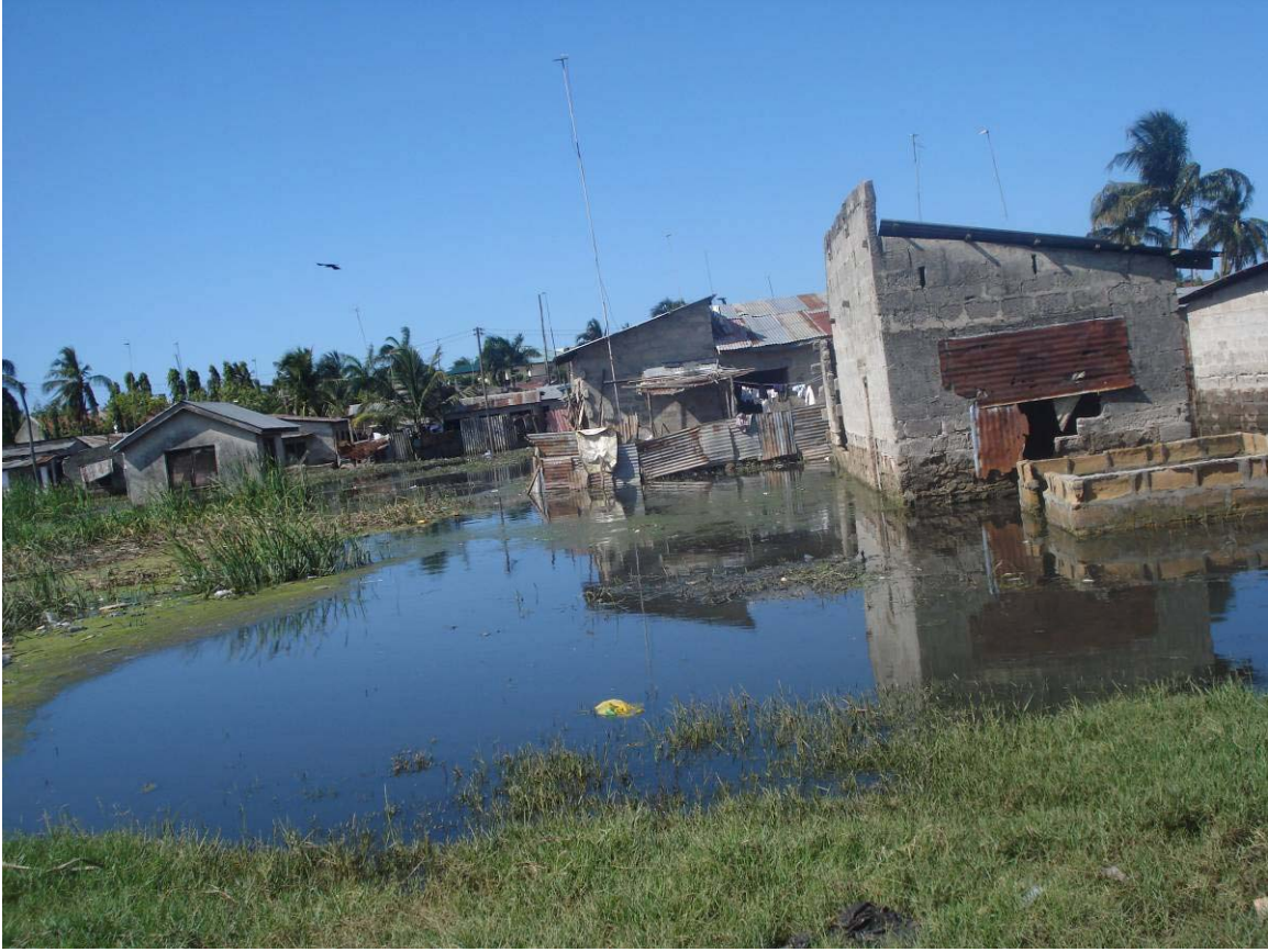
Plate 3.2: Flooded houses in the Bonde la Mpunga area during the rain season
