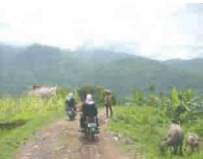
Rugged road condition
