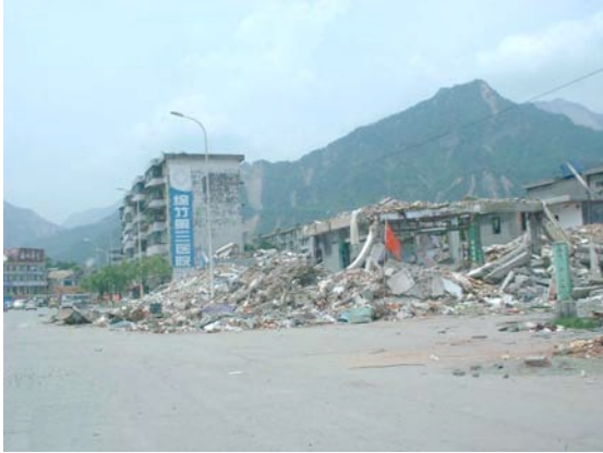
City center and mountain (Sloping failure)
