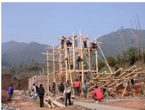
Traditional wooden house under reconstruction (in December 2008)
