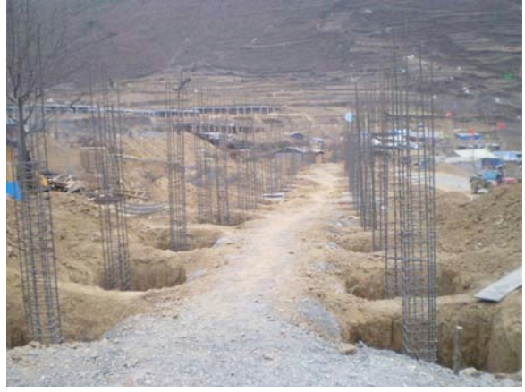
Construction halted due to cold (In Wenchuan, December 22, 2008)
