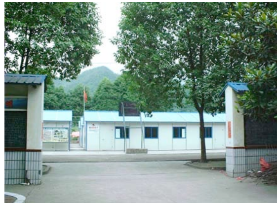
temporary elementary and junior high school in Zhundao Town (use of a ground of an elementary school)
