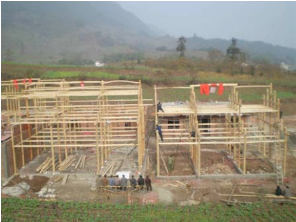
Housing reconstruction of wooden buildings (In Beichuan County, December 19, 2008)
