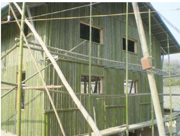
Housing reconstruction using bamboo by a Taiwanese architect (Beichuan County, December 24, 2008)
