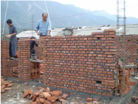
Housing reconstruction with brick and block (in Beichuan County, early October)
