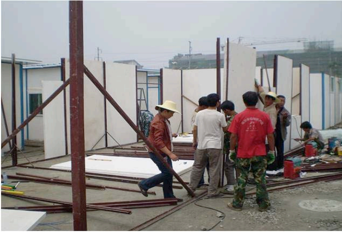
Temporary housing under construction (Dujiangyan City, June 23, 2008)
