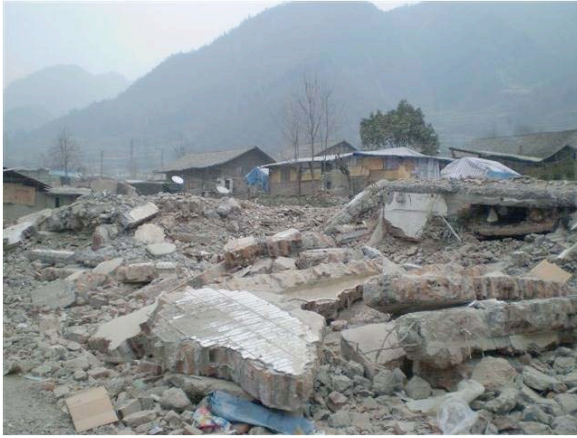
Left rubble, delay in support (In Wenchuan, December 22, 2008)
