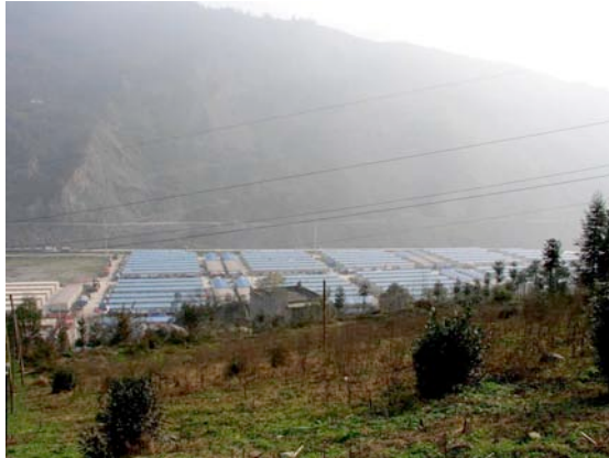
Temporary houses of Yingxiu Town of Wenchuan County
