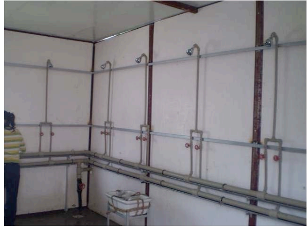
Shared shower room (Dujiangyan City, June 23, 2008)
