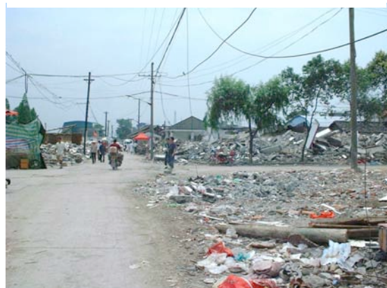
Piles of rubble of the city center, which almost totally collapsed
