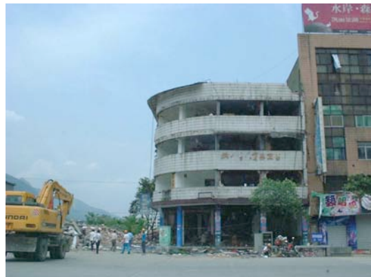
Removal of a collapsed hospital
