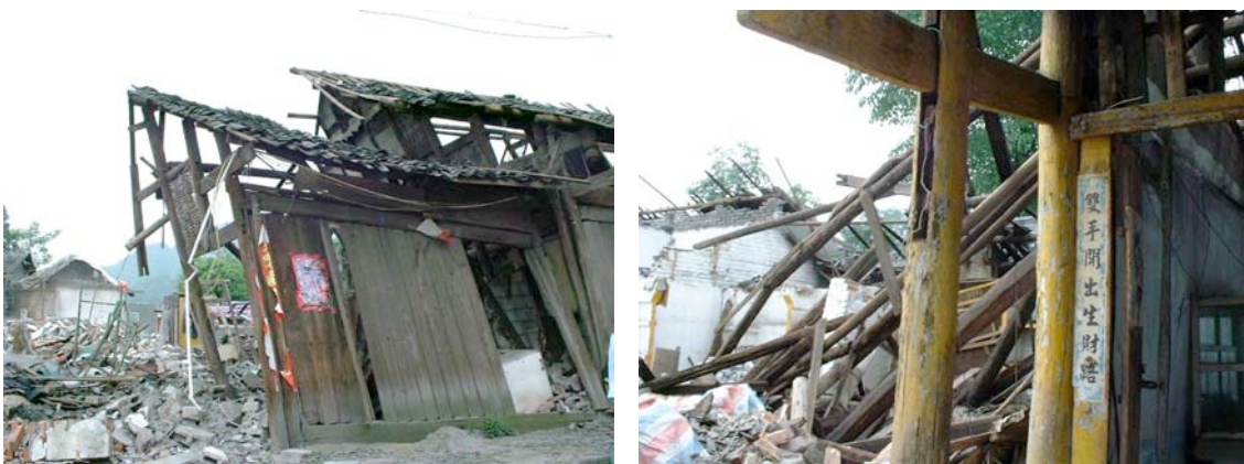
Damage on a wooden house in Zhundao Town of Mianzhu City (same for the right) Same framework method with columns and beams as in Japan. The photos were taken in June.
